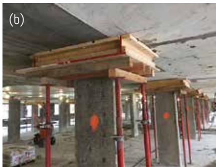
Fig. 4: Shear capital repair: (a) preparing and reinforcing the concrete surface, and (b) installed formwork prior to concrete pumping
