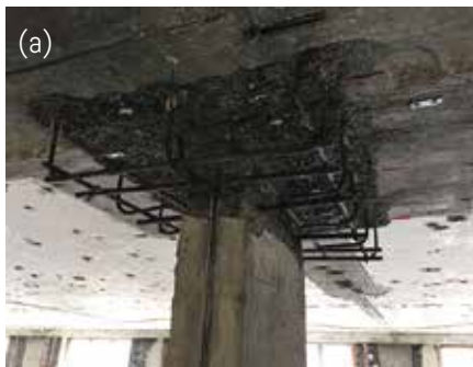
Fig. 3: Prepared slab around a column prior to installing the crack infill and CFRP
