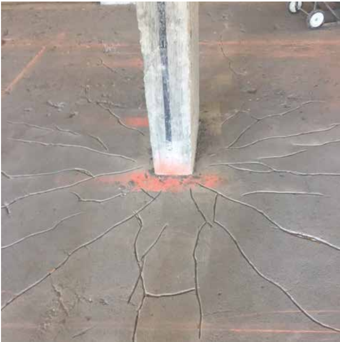
Fig. 3: Prepared slab around a column prior to installing the crack infill and CFRP
