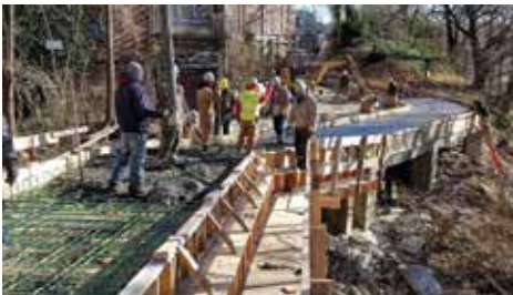
Fig. 7: Concrete placement at the pedestrian bridge
