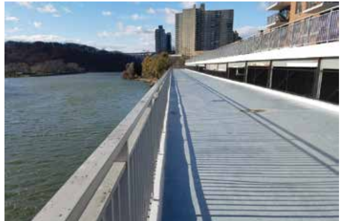
Fig. 3: Waterproofed promenade deck along the river
