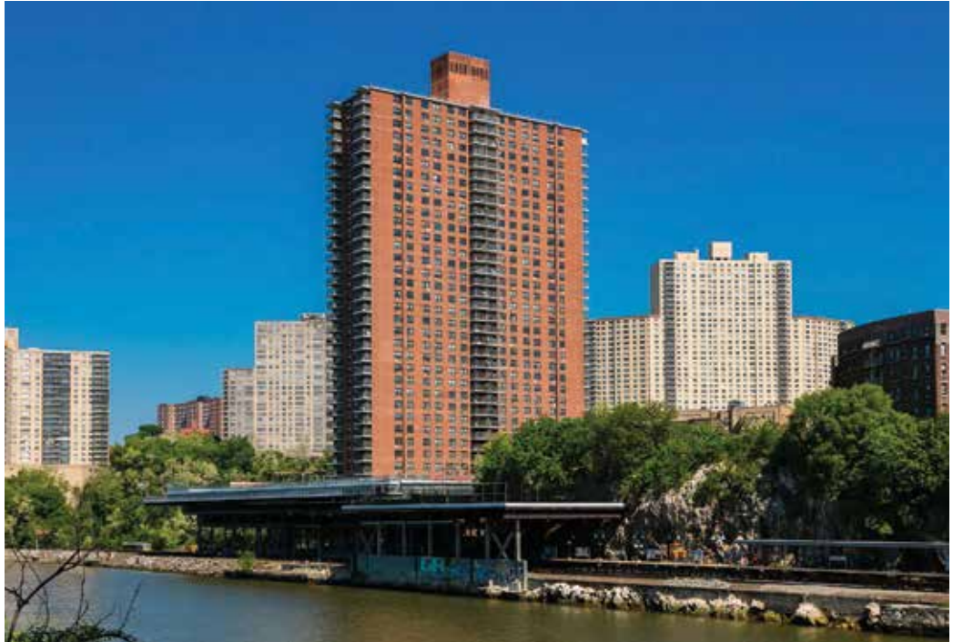
Fig. 1: The Promenade Apartment Building
