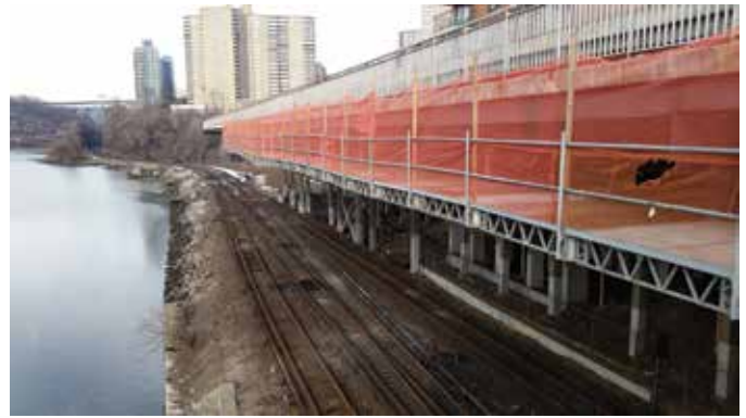
Fig. 2: Work platform suspended under the building
