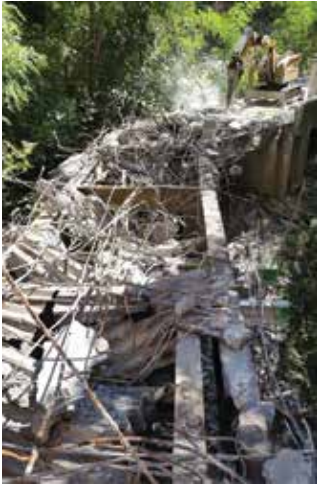
Fig. 6: Pedestrian bridge demolition
