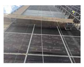
Damaging storms and prolonged exposure to the elements over many years in service subjected the façade to coating failure, caulking deterioration, corrosion of metal stucco corner beads and control joints, stucco cracking, and stucco delamination. In addition, prolonged water migration caused deterioration of the cold-formed steel wall studs supporting the façade and leakage into rooms. The reinforced concrete balcony slabs experienced cracking and spalling slab edges.
