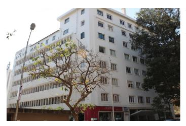
application of new sealants and coatings. The project consisted of repairs and replacement of major areas of the external façade, and repair to exposed portions of concrete elements, such as slab edges and columns. In addition, repairs included rehabilitation of the external façade treatment, replacement of façade render, repair/replacement of concrete members/slabs, jacketing of columns, corrosion control, and casting of concrete cornices and delicate architectural elements, including
