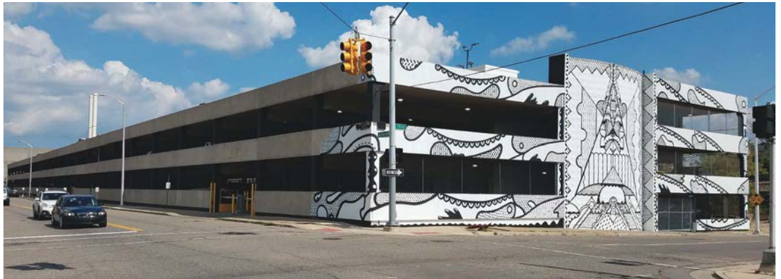
Fig. 1: Baltimore Parking Garage after repairs and showcasing a new exterior mural
