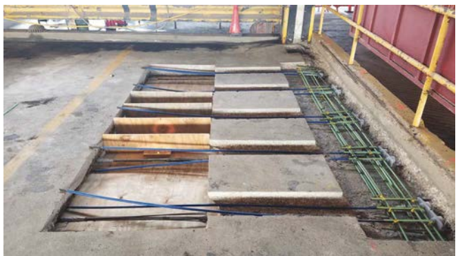
Fig. 4: Placement of new PT anchors
