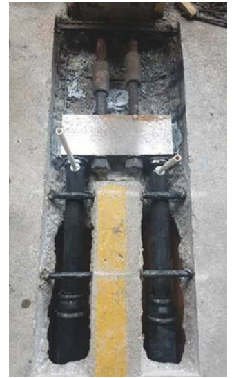
Fig. 6: External PT beam repair prior to running tendons through conduit
