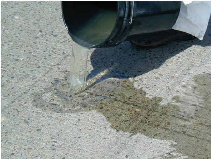
Fig.3: Pouring low-viscosity material into crack
