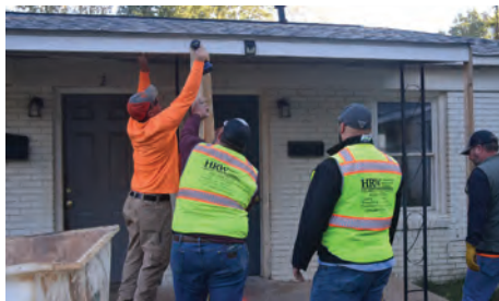
The work continues
