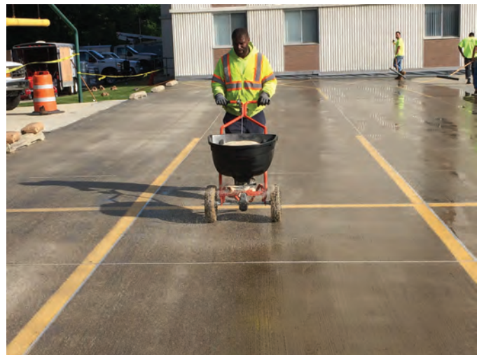
Fig. 5: Applying sand to material on deck slab
