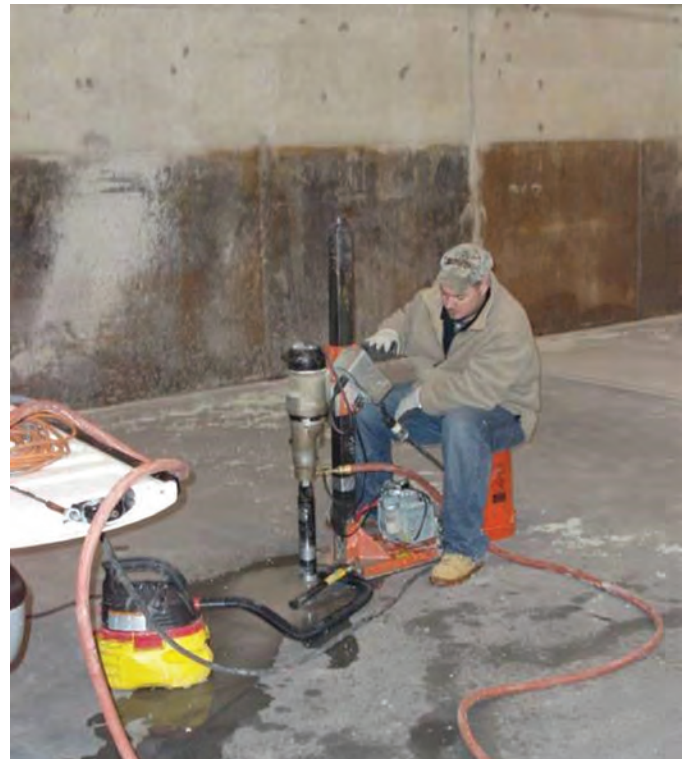
Fig. 2: Obtaining core specimens to determine compressive strength of concrete
