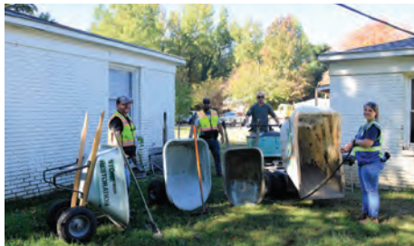
Preparing to wheel in the concrete
