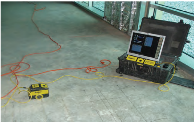
Fig. 4: Ground penetrating radar (GPR) to identify and verify locations of embedded reinforcing steel
