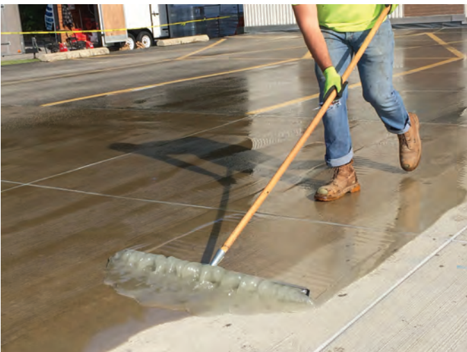
Fig. 4: Spreading material over deck slab
