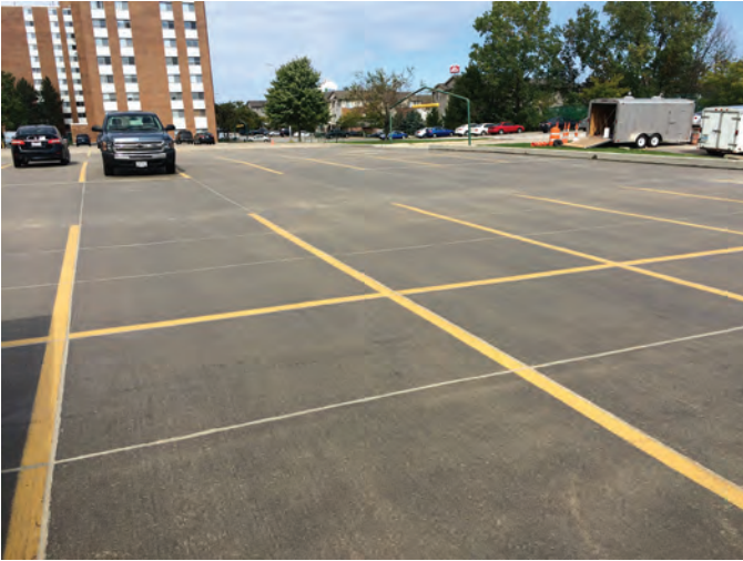
Fig. 6: Finished application on parking deck slab
