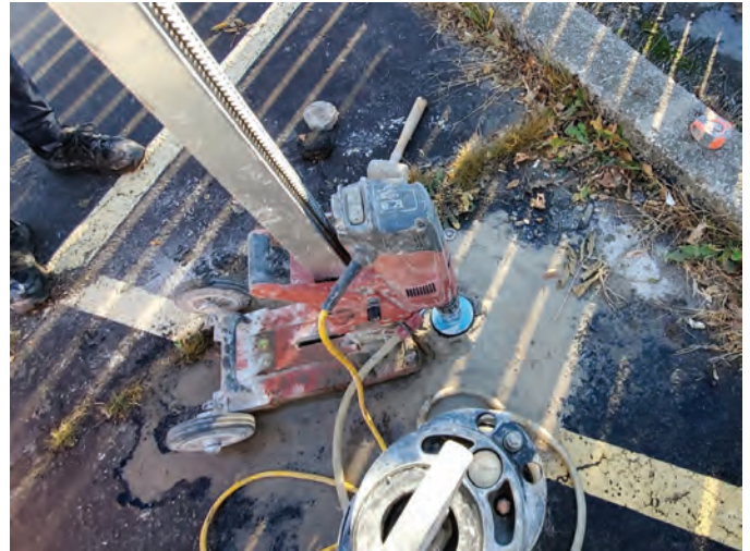
Fig. 6: Concrete core extraction for chloride testing at a garage roof slab
