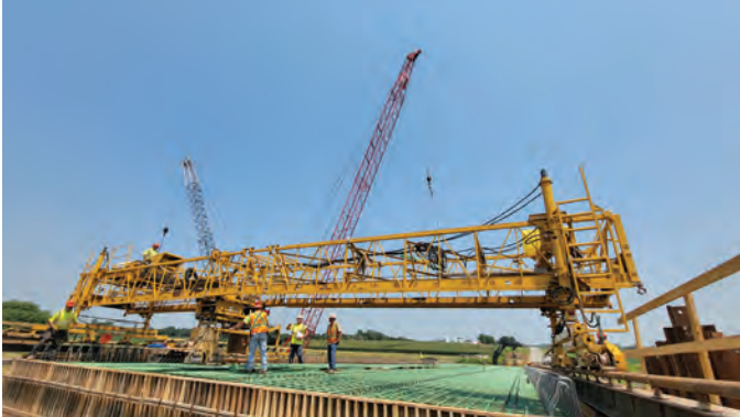
Field placement of UHPC on bridge (photo courtesy of Steelike)
