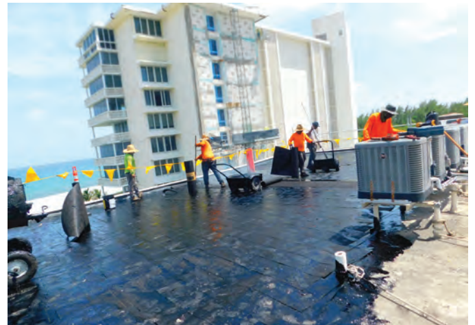
Fig. 6: The roof was replaced with a new built-up asphalt roof
