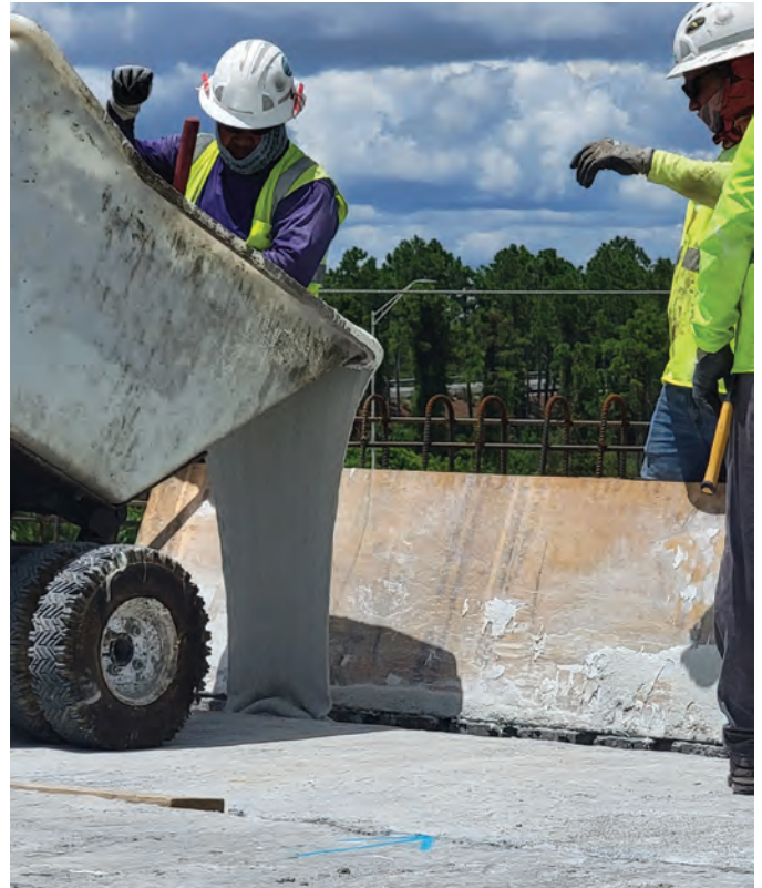
Field placement of UHPC (photo courtesy of Steelike)
