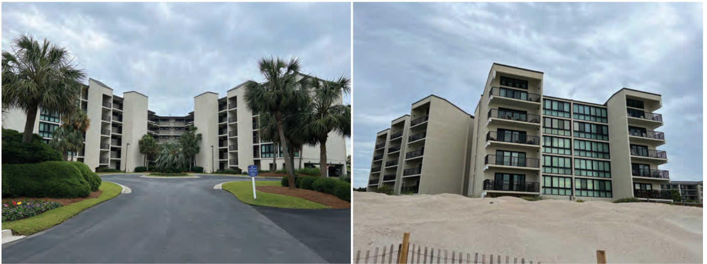
Fig. 1: 2023 photos: courtyard side of Building A (left) and ocean side (right)
