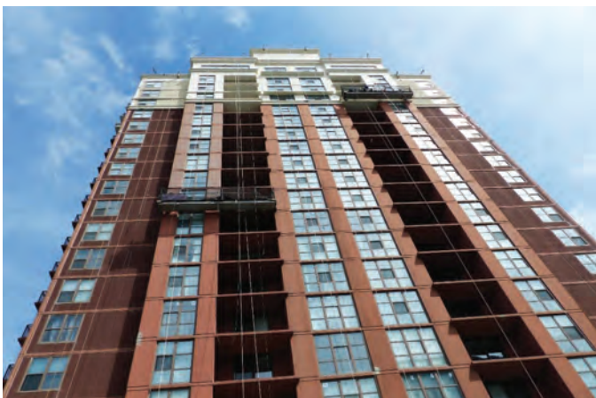
Fig. 8: Swing-stage work on south elevation
