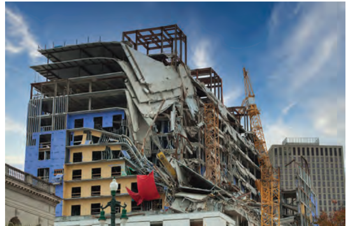
Fig. 2: Collapsed concrete slabs in a steel structure (Photo: BJ&C, www.bjc4ga.com)
