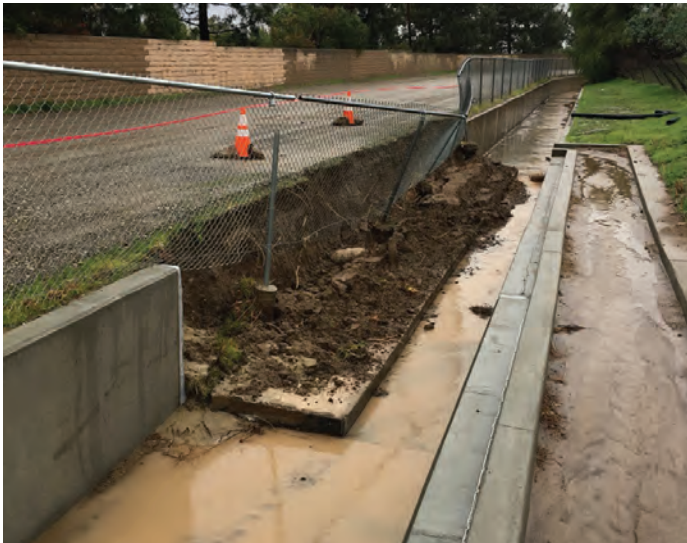
Fig. 1: Wall failures within two different channels.
