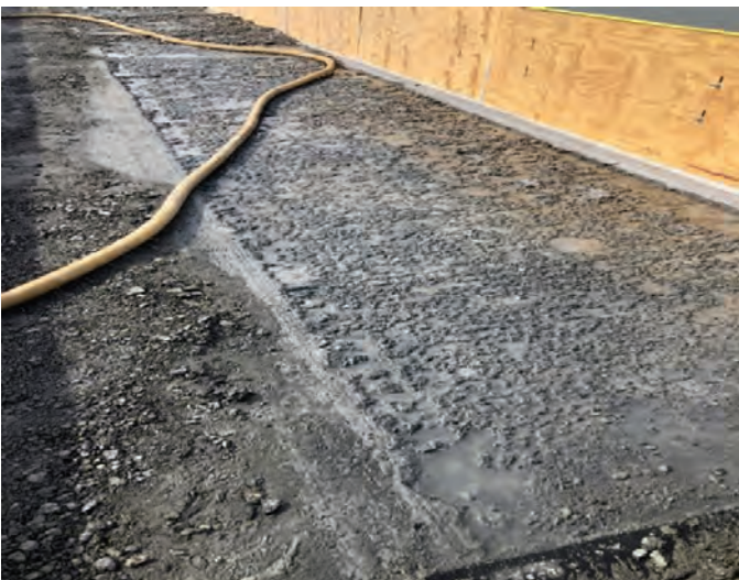
Fig. 5: Deck overlay substrate preparation by hydro-demolition (photo courtesy of SK&A)
