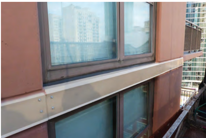
Fig. 7: Slab edge cover at east elevation
