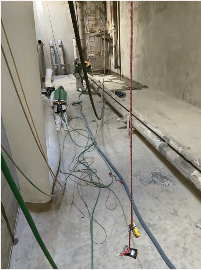
Fig. 11: Preparing to blast in tank
