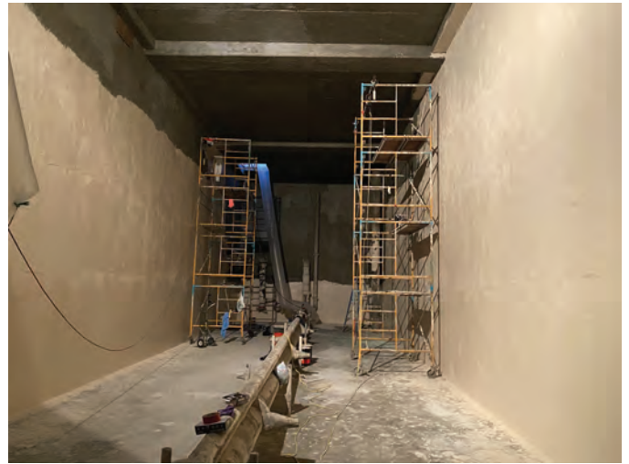
Fig. 12: Partially completed coatings in tank
