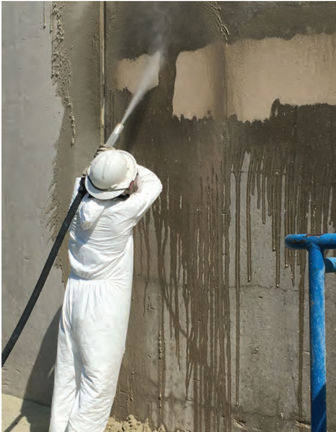
Fig. 7: Wet abrasive blasting with reduced dust emissions
