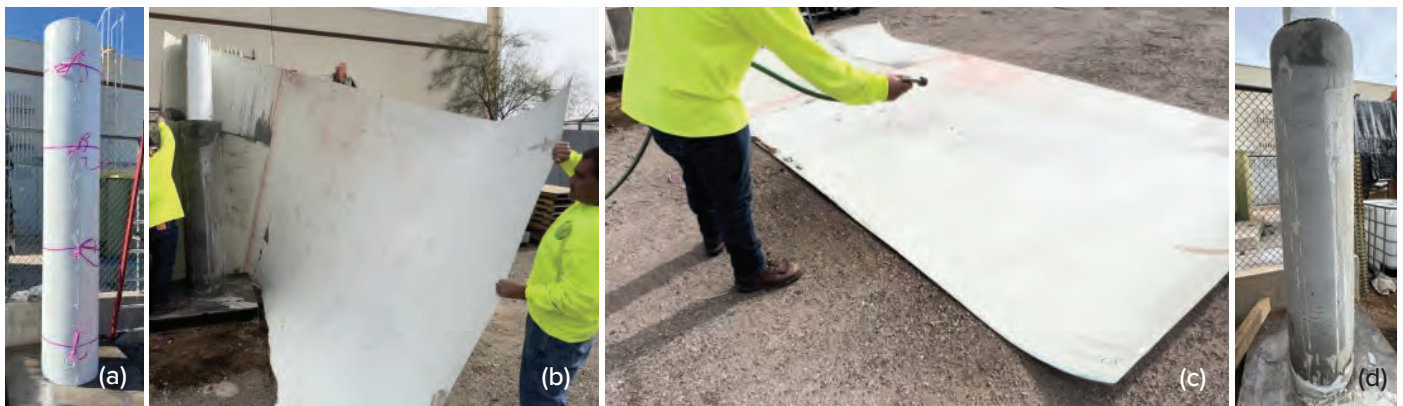
Fig. 3. Field application: (a) FLF placed and filled with concrete, (b) removing the laminate after concrete hardens, (c) cleaning and saving the laminate for future use, and (d) smooth concrete finish with no spiral marks
