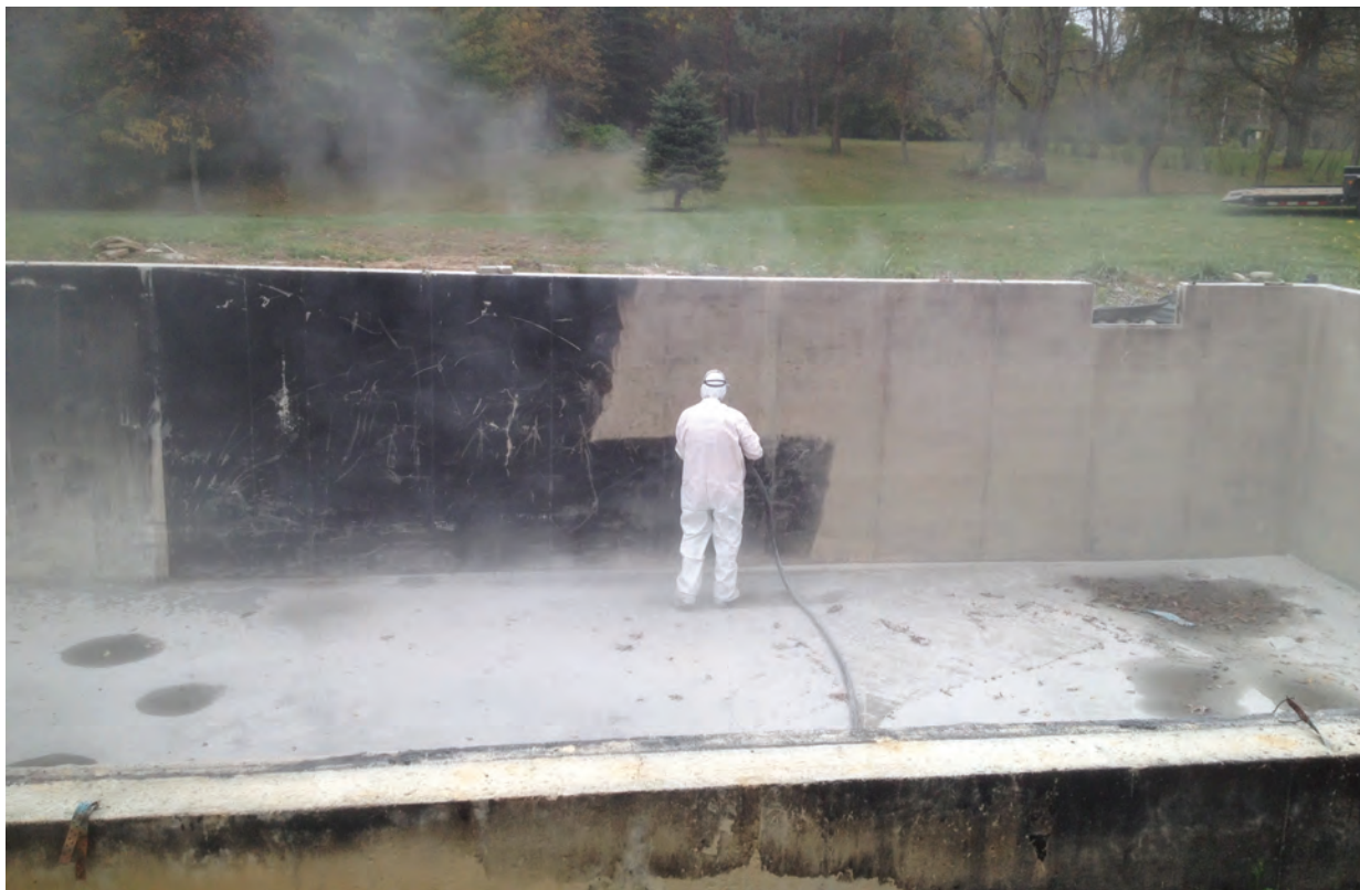
Fig. 1: Cleaning smoke residue with baking soda blasting
