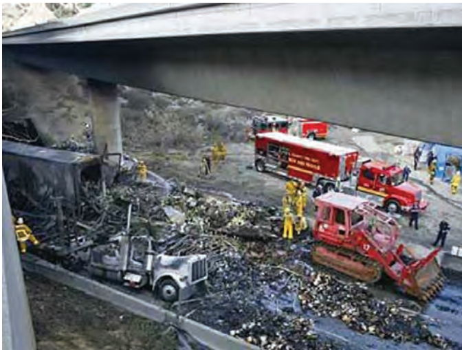
Fig. 2: It took approximately 24 hours to completely extinguish the fire. Photo source: Wiss, Janney, Elstner Associates, Inc.
