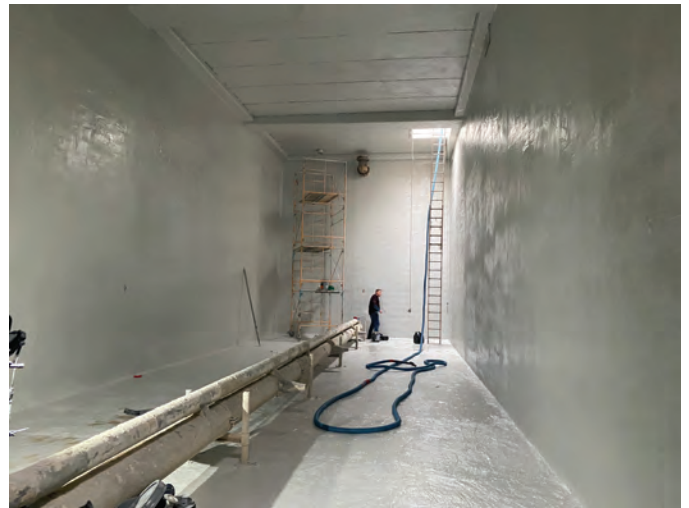
Fig. 13: Finished equalizer tank with all coatings applied
