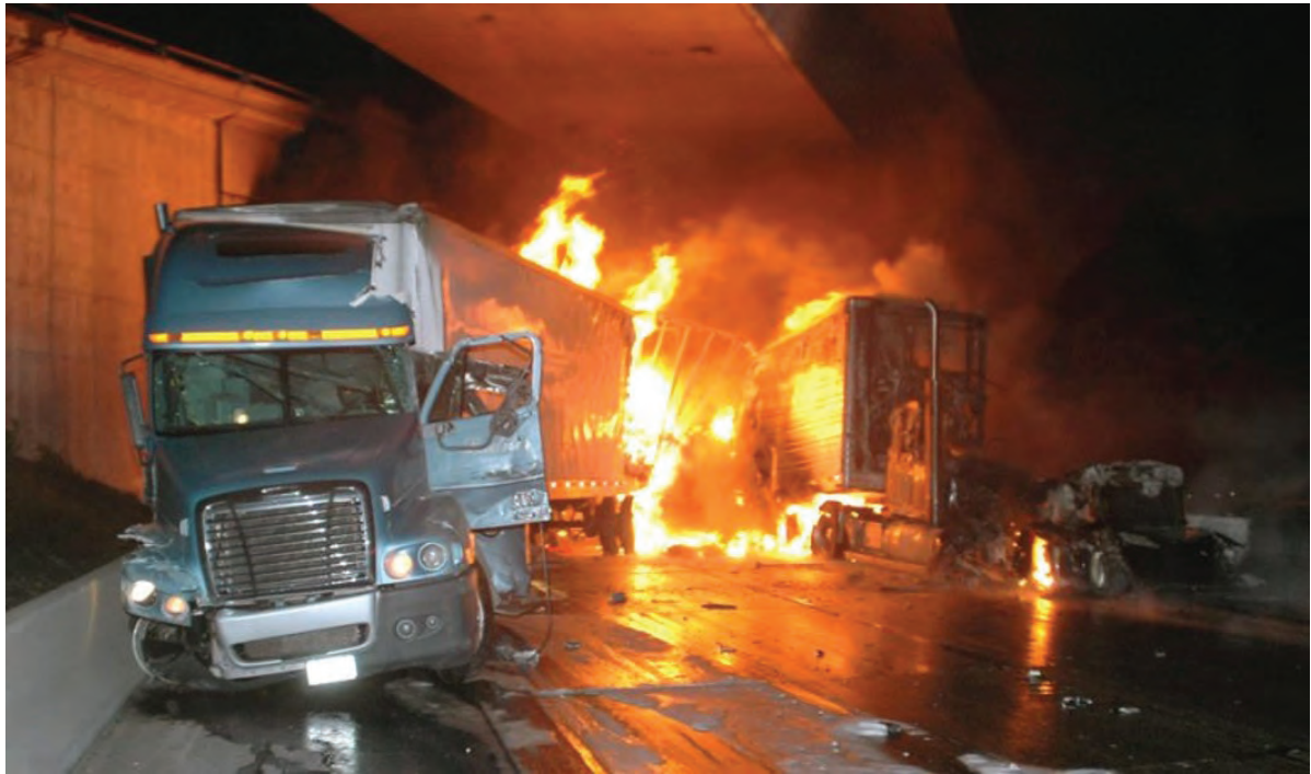
Fig. 1: The fire started on the evening of 12 October 2007 in a southbound Truck Bypass Tunnel that crossed under all lanes of I-5. Photo source: Wiss, Janney, Elstner Associates, Inc.
