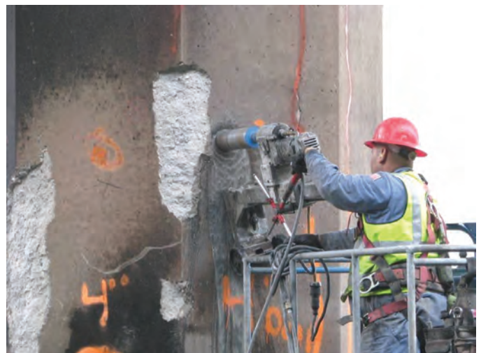
Fig. 6: 103 concrete samples were extracted from the undercrossing and examined in WJE laboratories in Illinois, Texas and Ohio. Photo source: Wiss, Janney, Elstner Associates, Inc.
