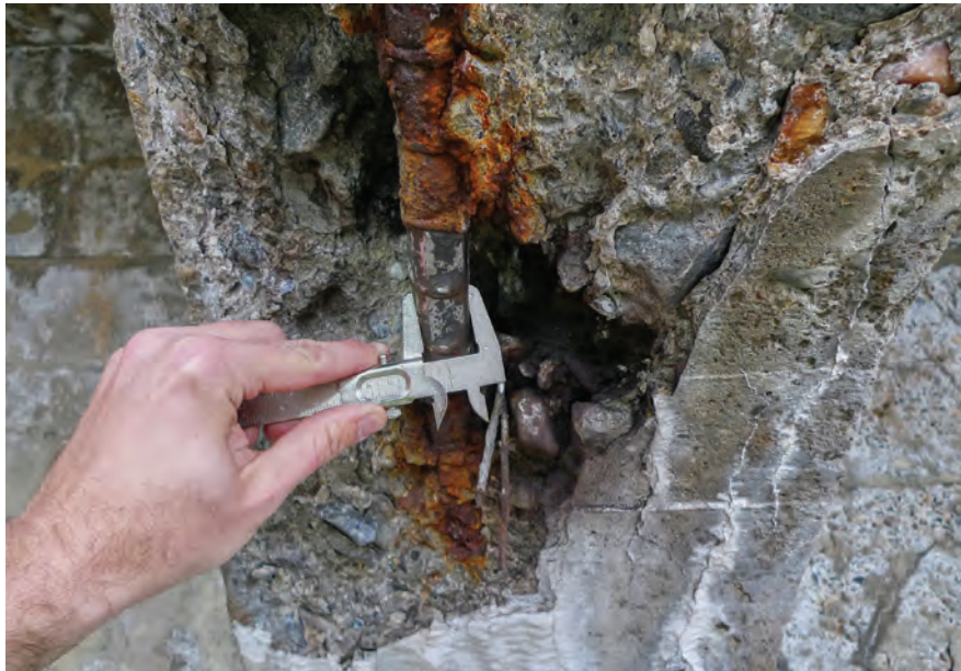
Fig. 1: Deformed, square cross section of reinforcing bar
