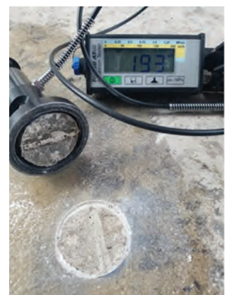
Fig.6: Performing ASTM D 7234 pull-off adhesion test
