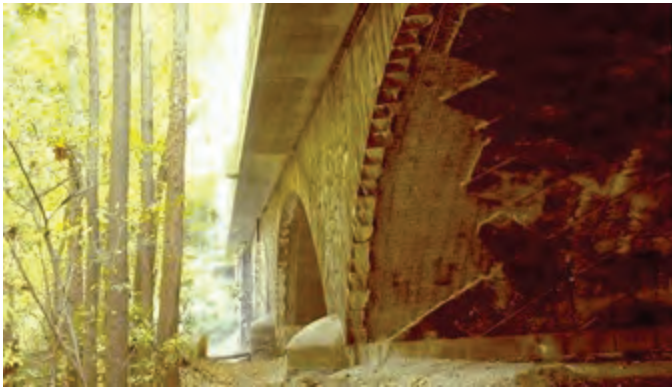
Fig. 5: Rehabilitation work on a concrete arch bridge (courtesy of D.W. Fowler)
