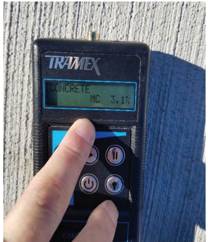
Fig. 1: Using an electronic non-destructive moisture meter
