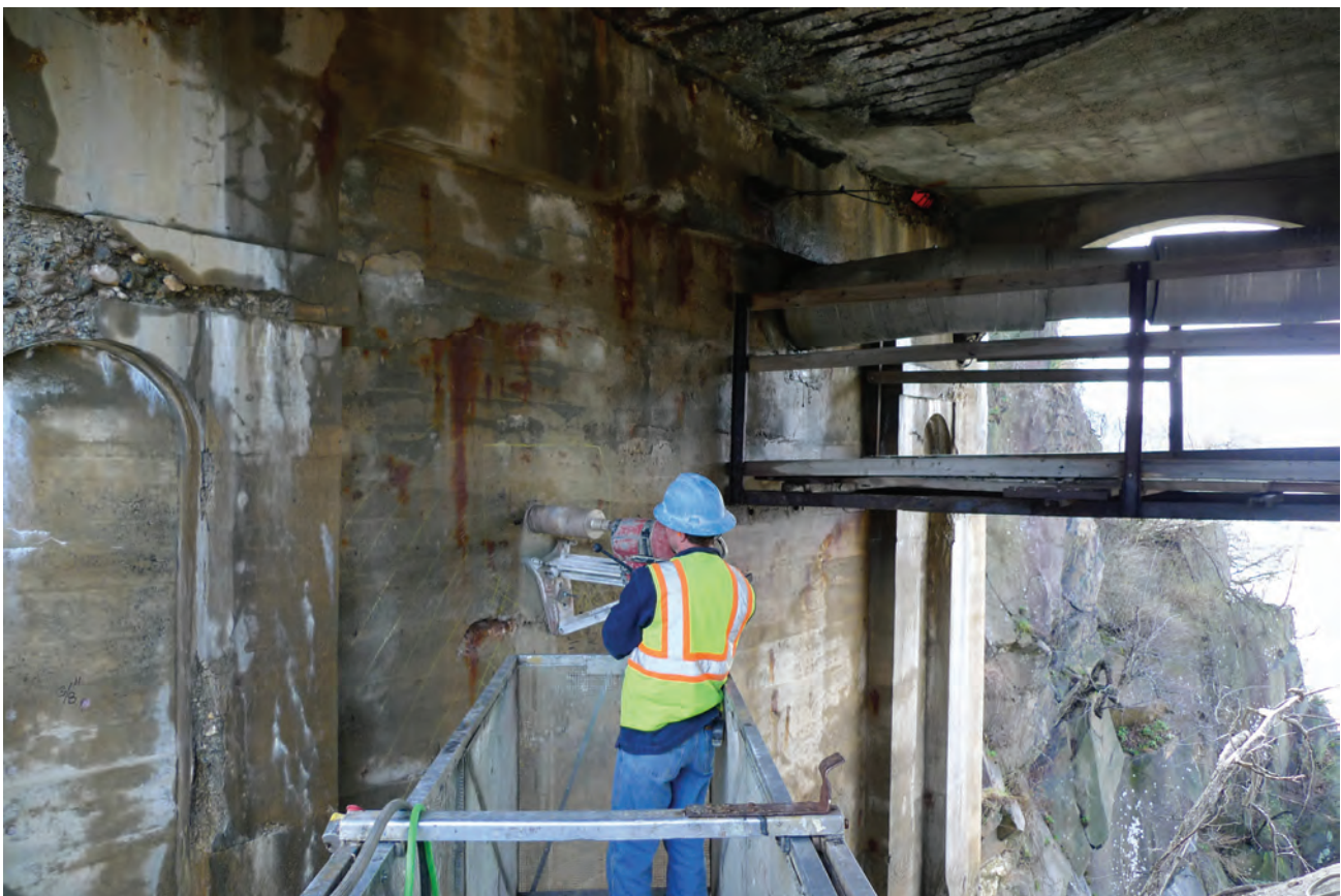
Fig. 1: Concrete core sampling for compression testing
