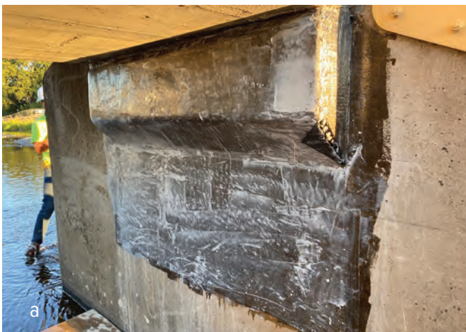
Figs. 3a and 3b: Carbon FRP was installed over the repaired corbel to extend the life of the structure and assist in preventing future deterioration
