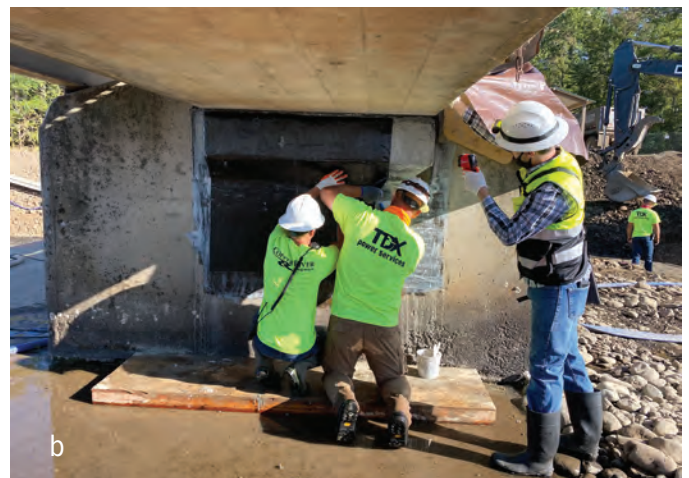
Figs. 3a and 3b: Carbon FRP was installed over the repaired corbel to extend the life of the structure and assist in preventing future deterioration
