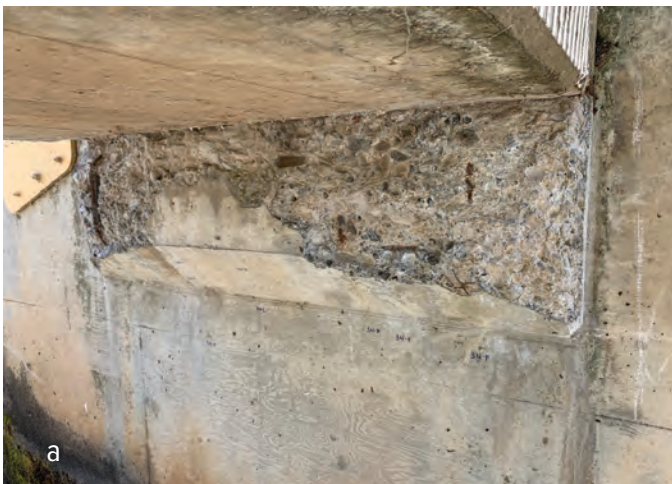
Figs. 2a and 2b: The corbel was deteriorated beyond what was expected, creating significantly more repair work prior to FRP installation
