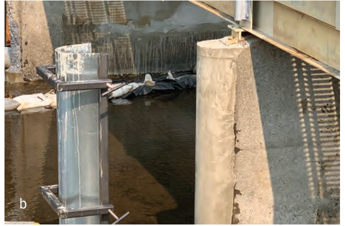
Figs. 4a and 4b: The contractor fabricated custom forms to enable access to the repair area for application of the epoxy bonding agent and speedy pour of rapid-hardening form and pour mortar
