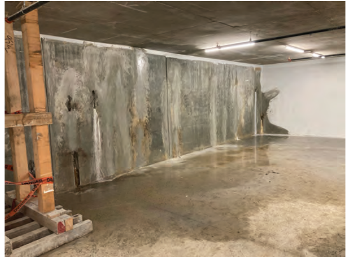
Fig. 2: Cast-in-place concrete structural walls with a crystalline grout application
