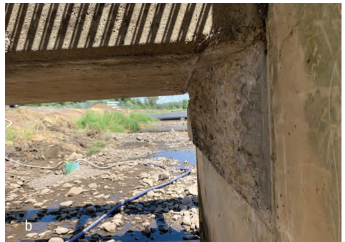
Figs. 2a and 2b: The corbel was deteriorated beyond what was expected, creating significantly more repair work prior to FRP installation
