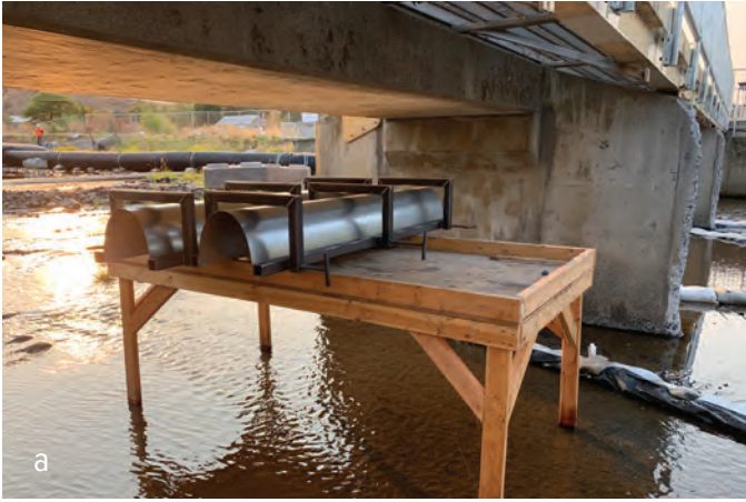
Figs. 4a and 4b: The contractor fabricated custom forms to enable access to the repair area for application of the epoxy bonding agent and speedy pour of rapid-hardening form and pour mortar
