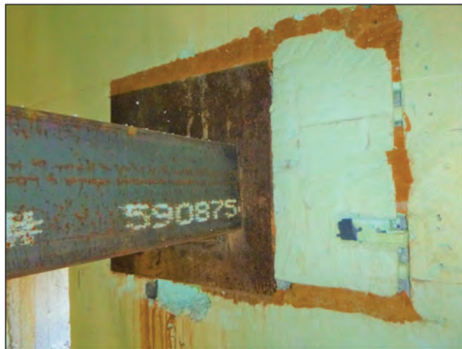
Fig. 9: Concealed concrete behind cast-in-place embed plate
