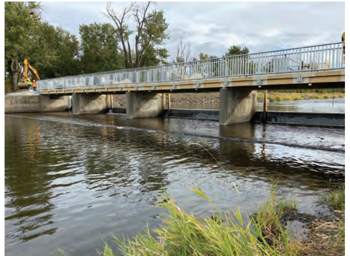
Fig. 5: Completed Project with damaged sections repaired, strengthened, and protected
