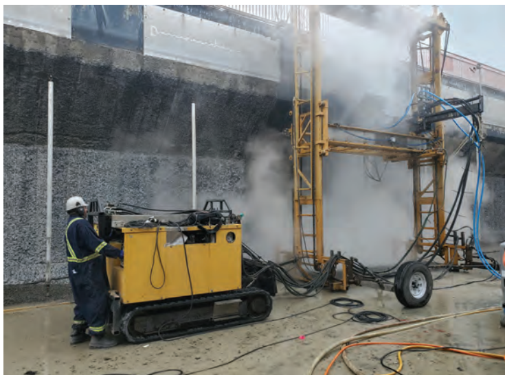
Fig. 3a: Custom hydro-demolition machine in usage
