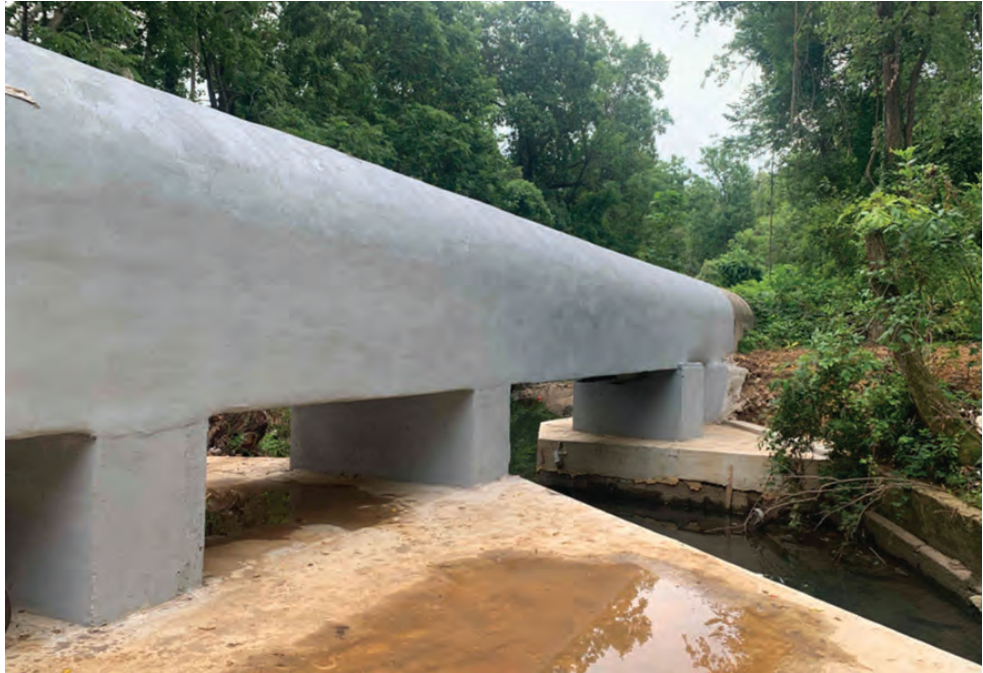
DC Water Aerial Sewer Crossing at the National Arboretum
