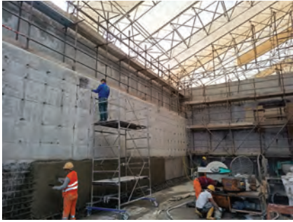
Fig. 9: Tank wall repairs and cathodic protection being installed
