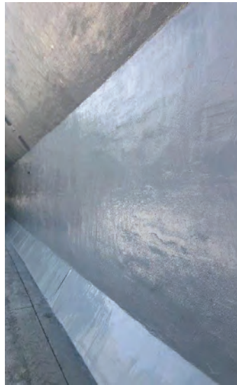
Fig. 5: Applied epoxy coating
