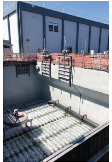
Fig. 6: Completed basin repairs in usage
