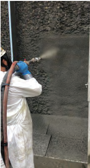
Fig. 4a: Shotcrete material actively sprayed
