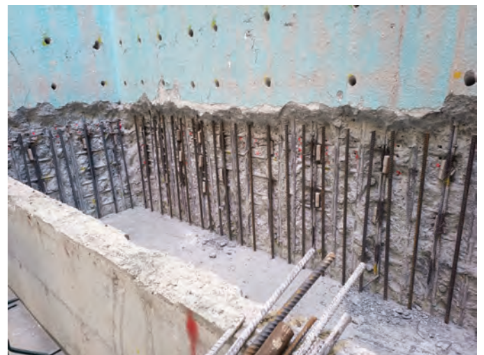
Fig. 8: Tank wall repairs with type 1A embedded galvanic anodes
