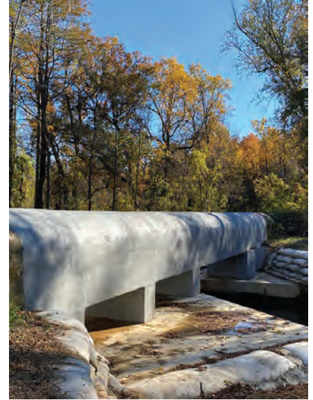
Fig. 6: The left-side view of the completed aerial sewer crossing
