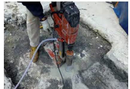
Fig. 6: Concrete cores were extracted for chloride and carbonation testing
