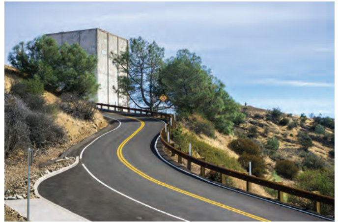
Fig. 6: Extremely steep road leading to the Radar Tower was the only way up or down
