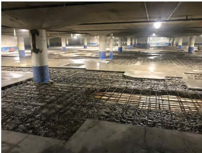
Fig. 6: Concrete surface preparation prior to placement
