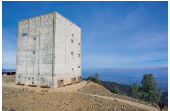
Fig. 2: Radar tower prior to asbestos remediation
