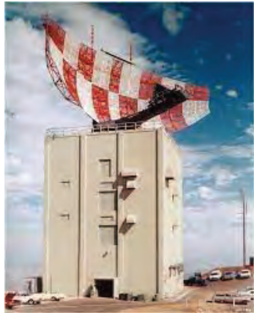
Fig. 1: Original photo of the radar tower with the radar still operational
