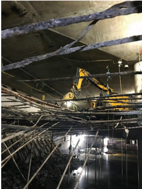
Fig. 5: Full-depth slab removal with remote-controlled robotic equipment (and lateral wall shoring)
