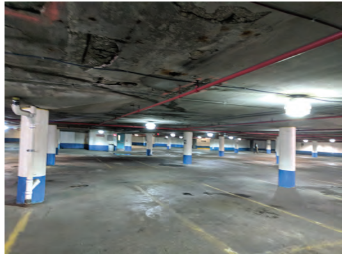
Fig. 1: Grand Circus Garage prior to renovation
