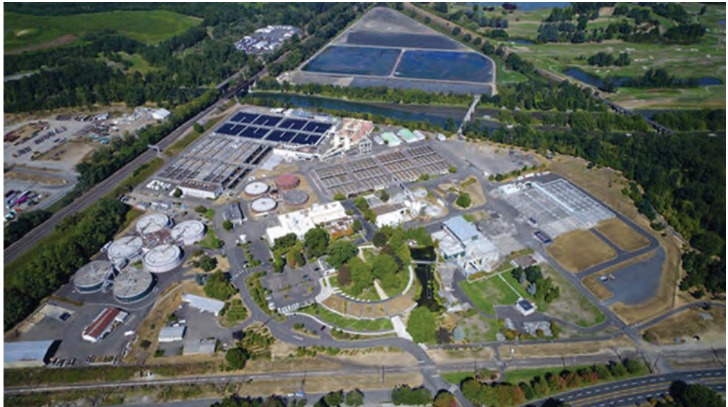
Columbia Boulevard Wastewater Treatment Plant
