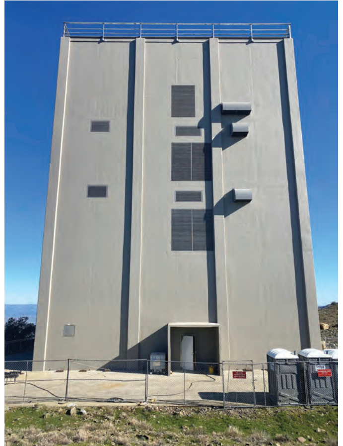
Fig. 10: Mount Umunhum Radar tower from the front
