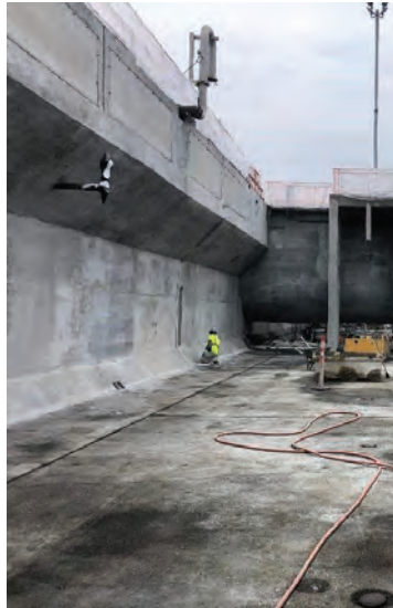
Fig. 4b: Completed wall application of shotcrete
