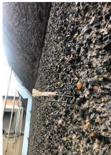
Fig. 3b: Post hydro-demolition wall surface
