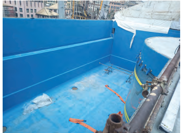
Fig. 12: Waterproof coating applied to mitigate future contamination
