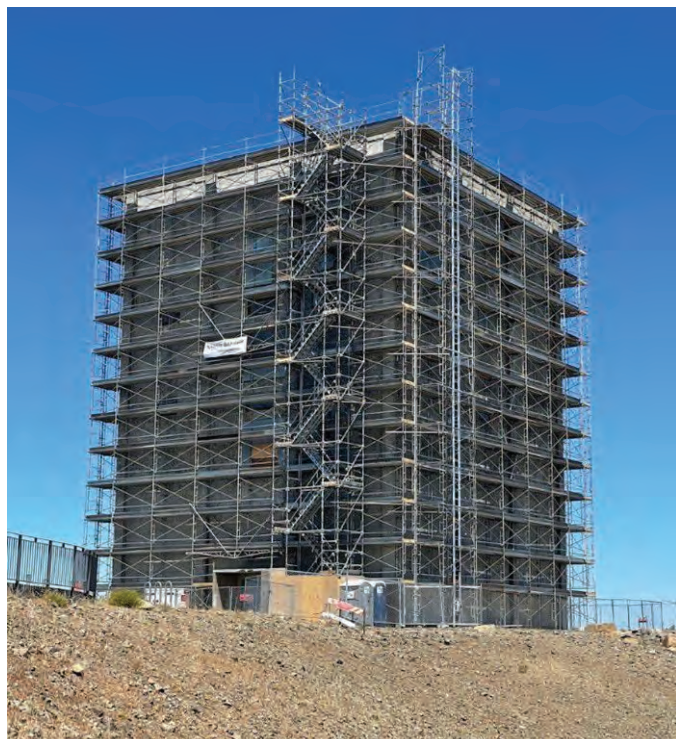
Fig. 5: Entire building scaffolded prior to repair work
