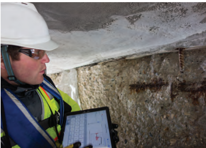
Fig. 3: Bridge inspector recording notes utilizing proprietary iOS-based tablet inspection software (photograph by WJE)
