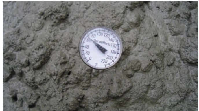
Fig. 3: Concrete placed at recommended temperature in cold weather conditions
