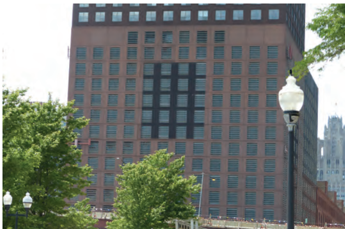
Fig. 1: East elevation louvers
