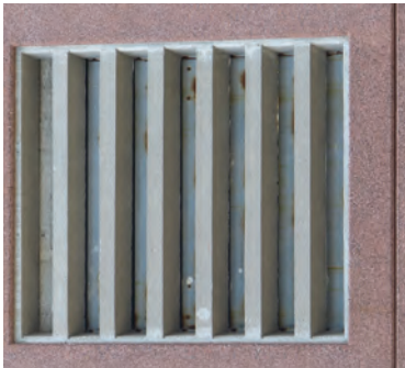
Fig. 3: Typical louver configuration
