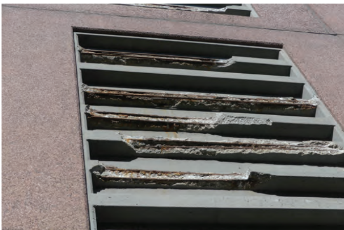
Fig. 9: Loose concrete removed periodically
