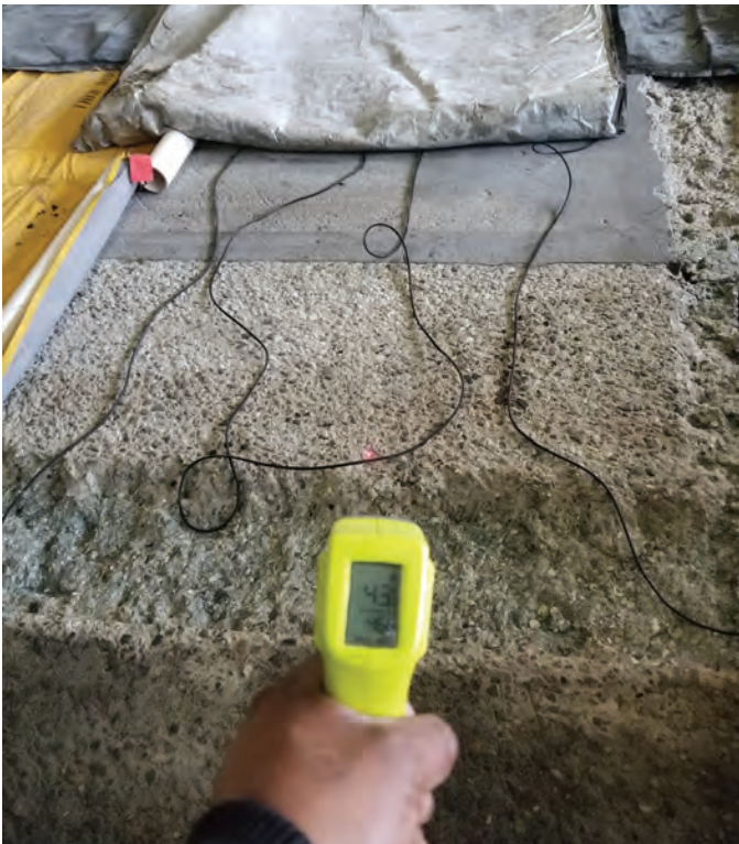
Fig. 7: Warming substrate with heated blankets, coils, and insulation
