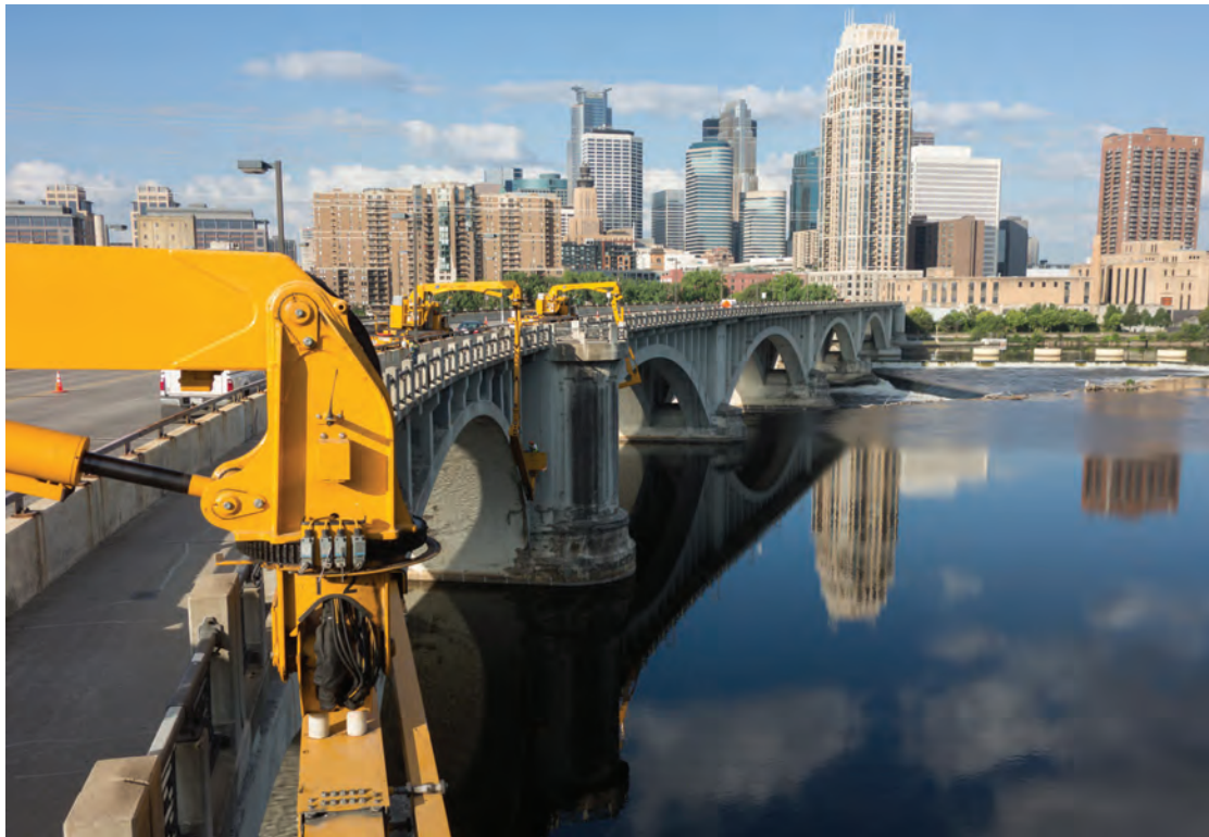
Fig. 1: Engineers utilizing three under bridge inspection units for close-up bridge inspection and sounding during the Phase 1 bridge inspection (photograph by WJE).
