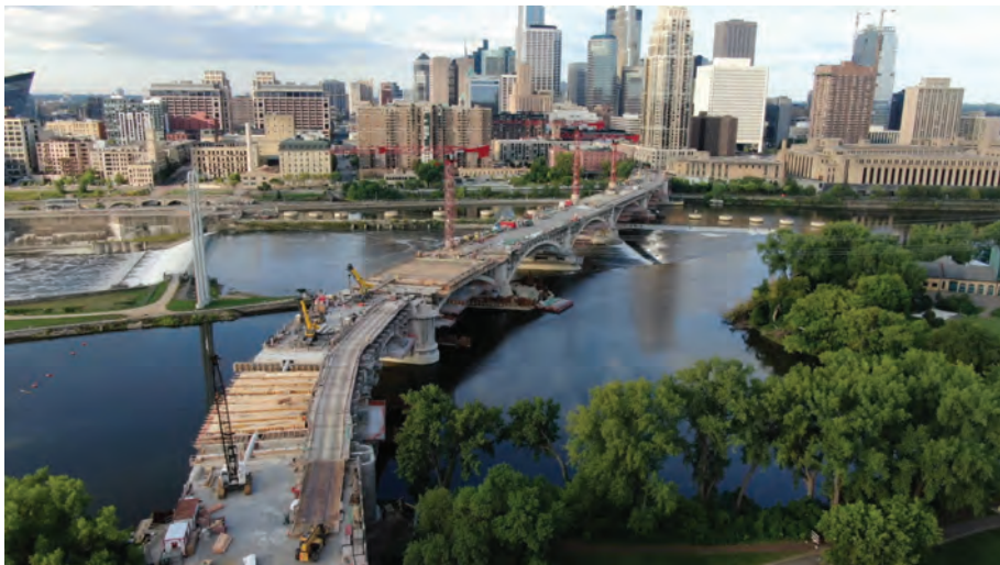
Fig. 9: Recent drone image showing status of the in-progress construction (photograph by WJE)
