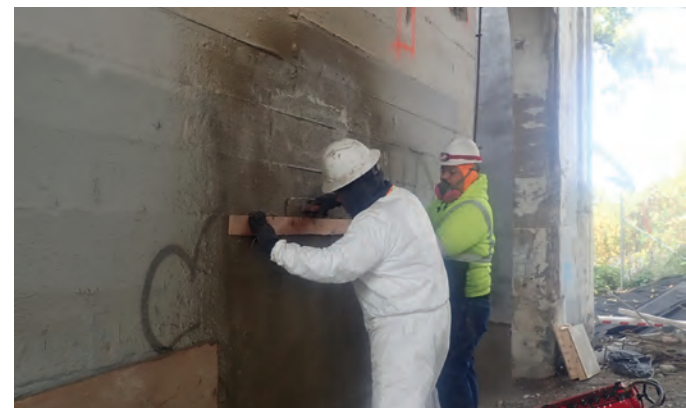
Fig. 8: Example of board-form finish achieved using hand floats in shotcrete surface repair (photograph by WJE).
