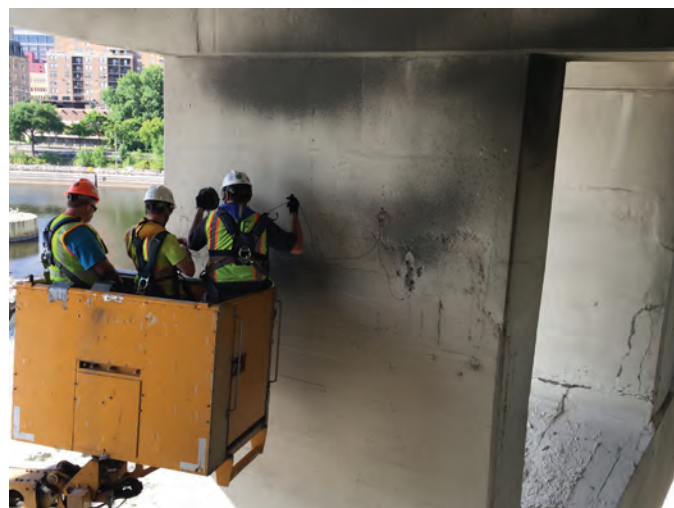
Fig. 2: Engineers utilizing three under-bridge inspection units for close-up bridge inspection and sounding during the Phase 1 bridge inspection (photograph by WJE).
