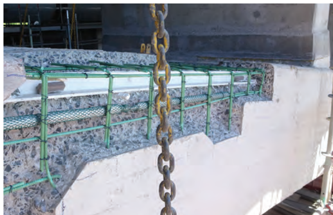
Fig. 6b: Arch corner repair prepared for concrete placement
