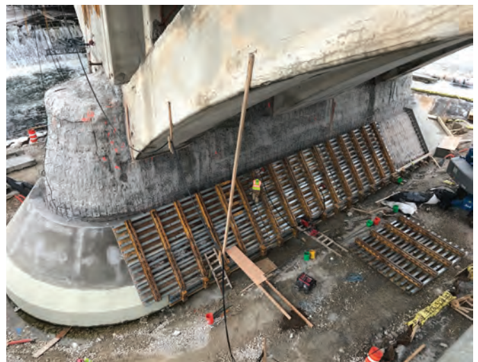
Fig. 5: Concrete removals completed, reinforcing steel being placed, and new pier jacket concrete being formed and placed (photograph by WJE)
