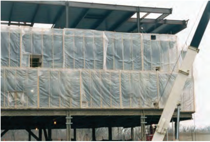
Fig. 5: Heated enclosures to create a temperature- controlled environment
