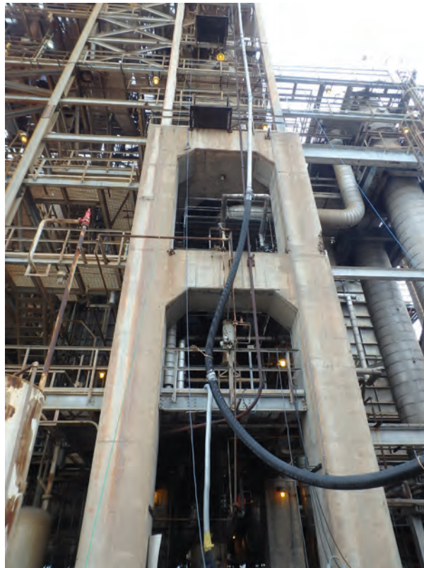
Fig. 1: Catalytic reformer support structure
