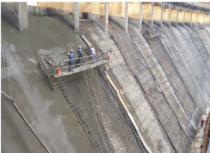
Fig. 6: Wet-mix shotcrete application
