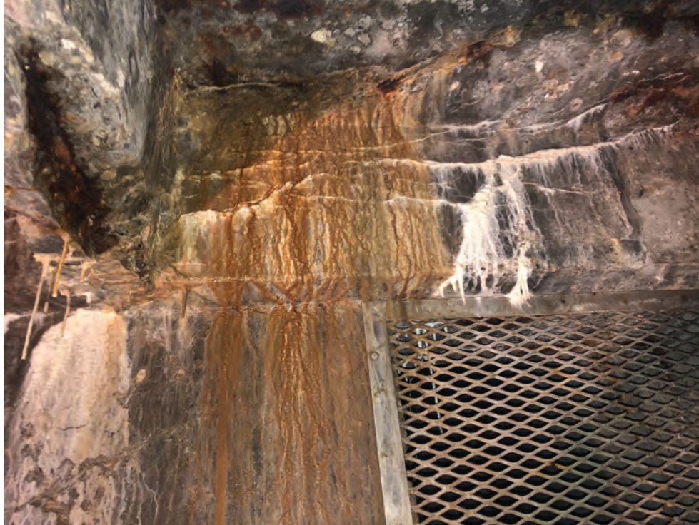
Fig. 1: Condition of a water treatment plant that was constructed in 1907
