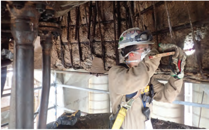
Fig. 6: Measuring depth of drilled hole used for chloride and carbonation testing
