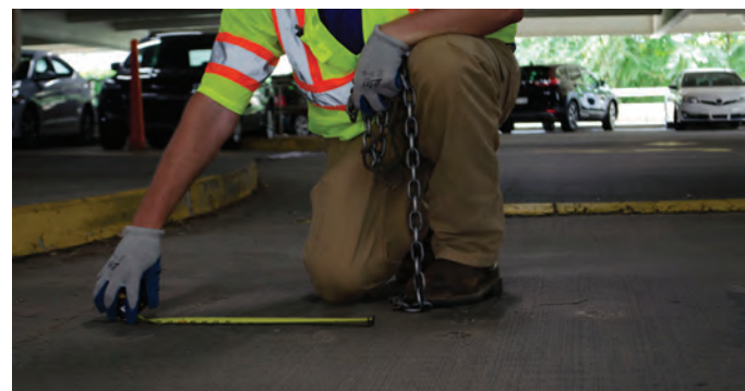
Fig. 3 Sounding using a chain drag
