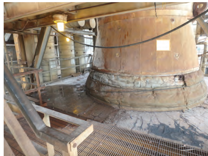
Fig. 5: Widespread cracking on top of upper deck, typically emanating radially from the catalytic reformer
