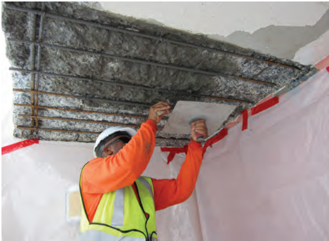
Fig. 4: Unformed hand-applied application
