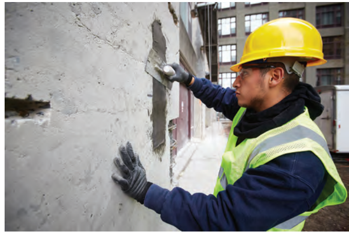
Fig. 8: Vertical surface repair creates composite with the existing concrete
