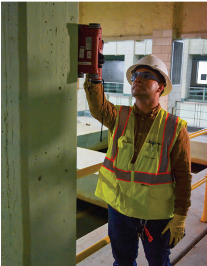
Fig. 4: Inspector using ferromagnetic rebar locating device
