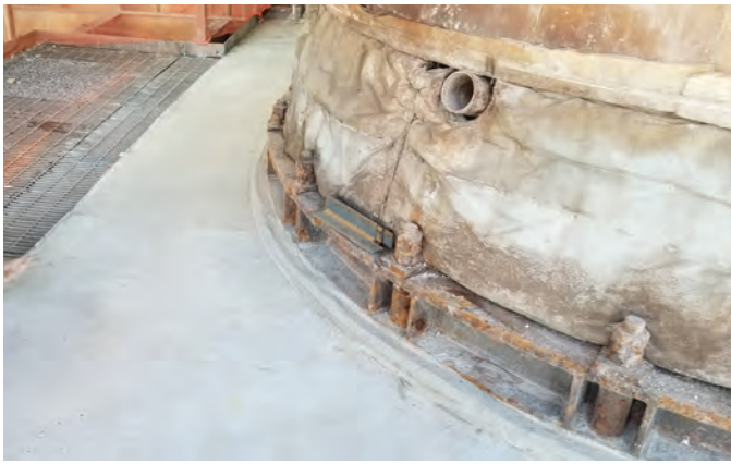
Fig. 12: Completed repair on top of upper deck
