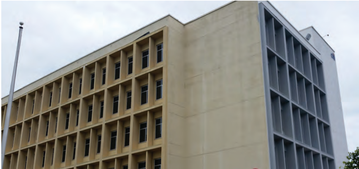
Fig. 1: 4-story bank building in Nassau, Bahamas
