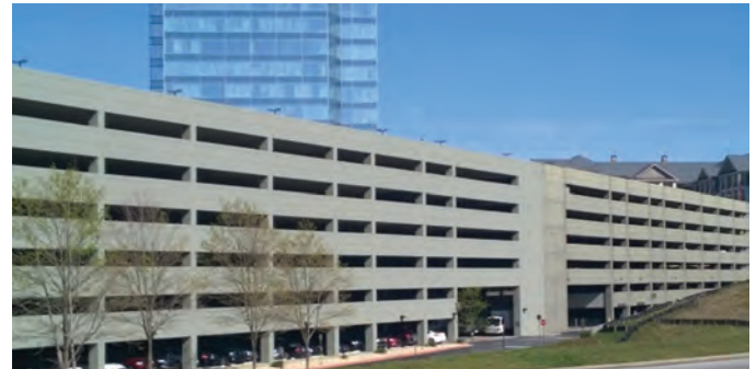
Fig. 10: Properly coated concrete parking structure
