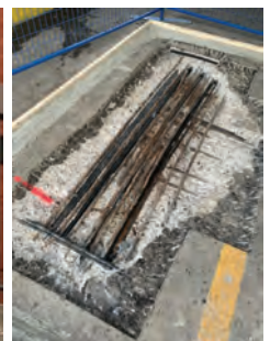
Fig. 8: Removal of unsound concrete in progress at PT strands
