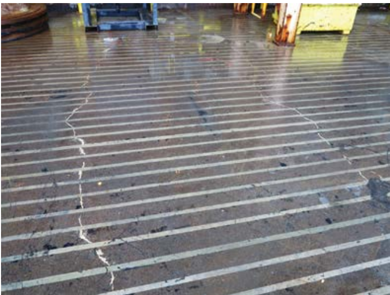
Slab strengthening and repairs completed
