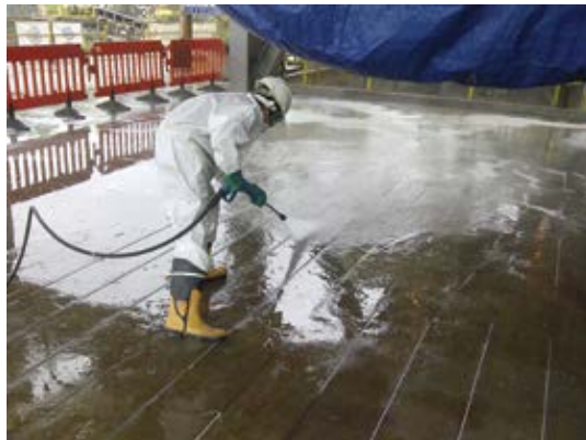
Water blasting CFRP slots
