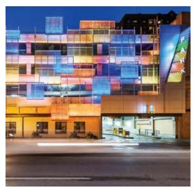
ocated between two government buildings in Lexington, KY, the Helix-on-Main parking structure, formerly known as the Annex parking structure, is a 1970s conventionally reinforced cast-in-place concrete parking garage with a helix ramp that was renovated and re-imaged to better serve its community.
