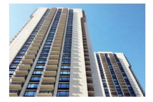
In the spring of 2015, both buildings were visually inspected from the ground and photographed using high-powered lenses. No signs of corrosion damage (cracking or spalling) were observed, and the remote monitoring confirmed this observation as all areas remained passive. The protective coating is still in good condition and the sealant, while generally in good condition, showed some signs of aging. Most importantly, the owner is very pleased with the performance of the project.
