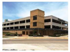
he University of Missouri Health Care Patient and Visitor Parking Structure (referred to as the MUHC Garage) was built in 1986 with a capacity of 448 vehicles. The MUHC Garage consists of three elevated post-tensioned (PT) concrete decks and a slab-on-ground.
