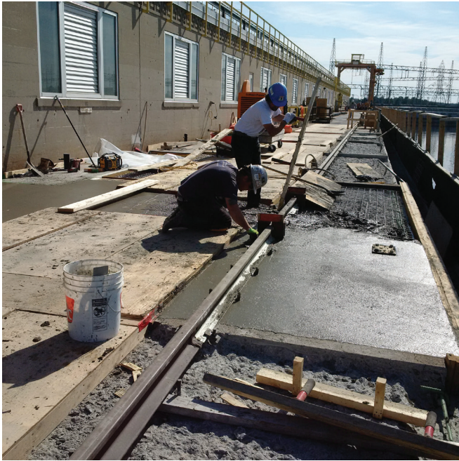
Fig. 5: Finishing deck concrete
