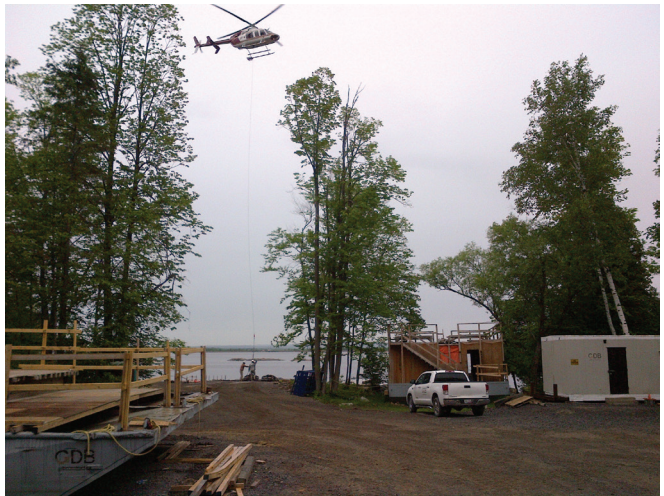
Fig. 2: Helicopter transports materials and equipment
