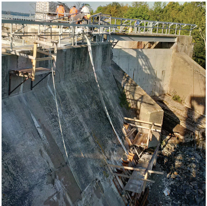
Fig. 3: Placing concrete into wall forms
