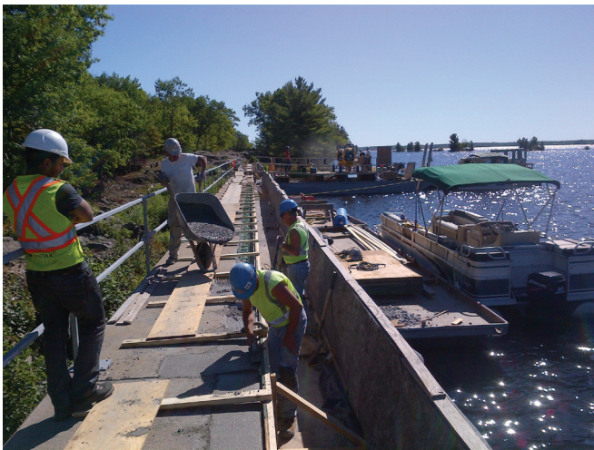
Fig. 6: Placing deck concrete
