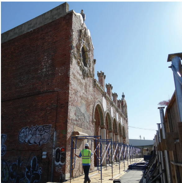
Fig. 6: Scaffolding was erected and re-erected numerous times throughout the project
