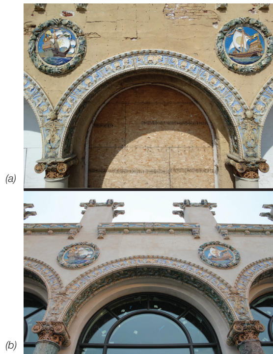
Fig. 4: (a) Terra cotta detail before, (b) and after
