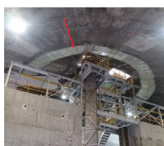
Fig. 8: GFRP strengthening system applied externally under upper stiffener ring
