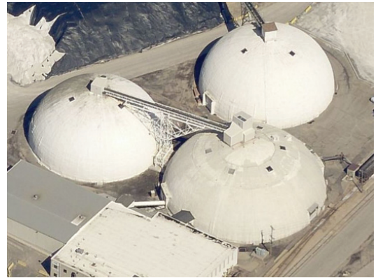
Fig. 1: Overhead view of salt storage and packaging facility
