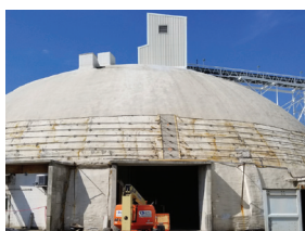
Fig. 7: Installation of new external post-tensioning system on dome above doorway eyebrows
