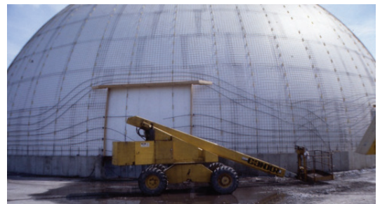
Fig. 2: Monolithic dome reinforcing during original construction prior to shotcrete placement
