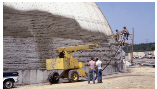
Fig. 3: Shotcrete placement over welded-wire fabric and post-tensioning tendons during original construction
