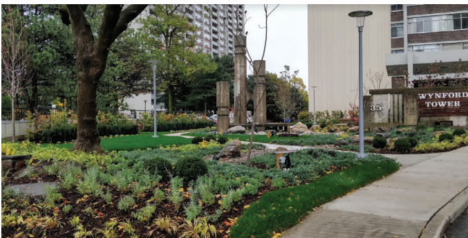
Fig. 7: Completed podium deck
