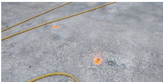
Fig. 3: Anodes installed in sound parent concrete where corrosion potential was high
