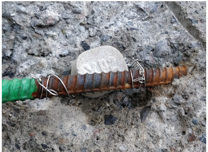
Fig. 2: Galvanic anodes inside a concrete repair area
