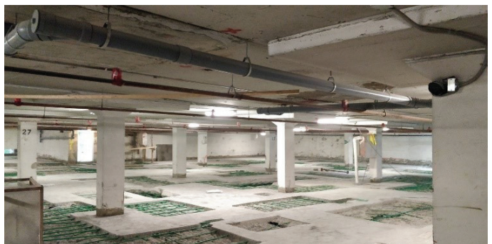
Fig. 4: Concrete repairs on intermediate slab
