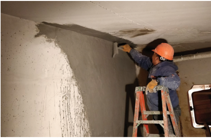
Fig. 5: Crystalline waterproofing the negative side of foundation wall
