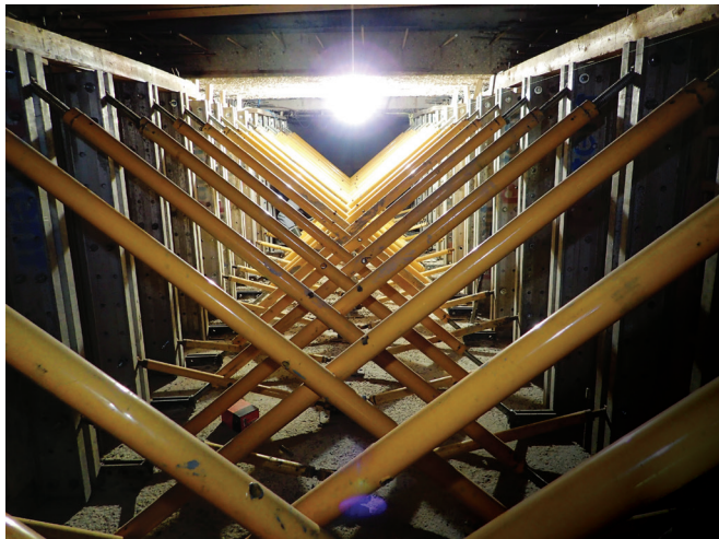
Fig. 6: Formwork and bracing
