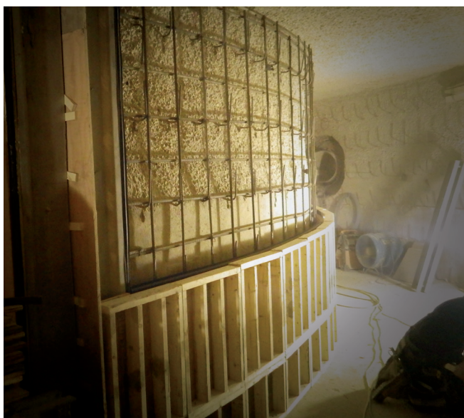
Fig. 5: Wall liner, reinforcement, and formwork
