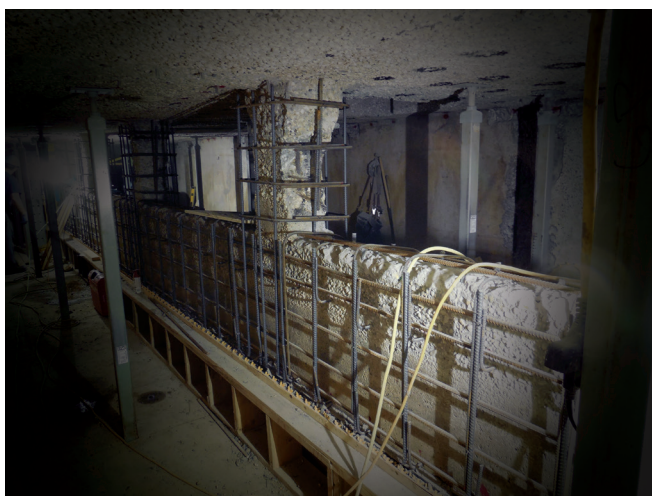
Fig. 4: Overlay reinforcement at overflow weir
