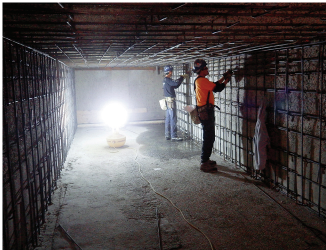
Fig. 3: Reinforcing installation within channel
