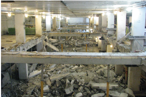
Fig. 6: Demolition and temporary lateral bracing in Phase 2
