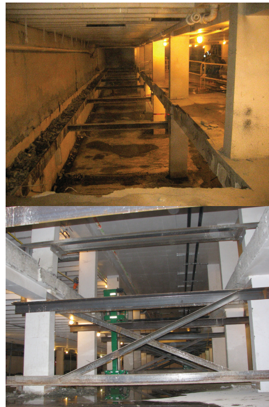
Fig. 4: Demolition and temporary lateral bracing in Phase 1
