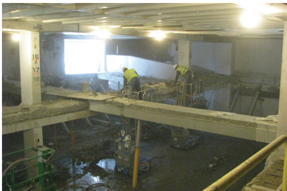
Fig. 8: Detail demolition during Phase 2
