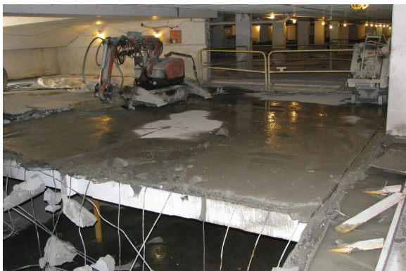
Fig. 7: Large-scale demolition during Phase 2
