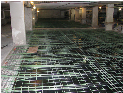
Fig. 10: Steel reinforcement for new pan-joist system (Phase 2)
