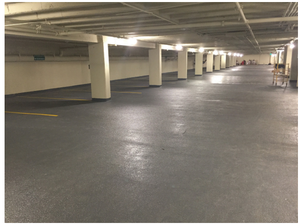
Fig. 11: Vehicular traffic-bearing waterproofing (VTBW) system installed on Level G1
