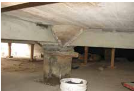
Fig. 8: Girders after concrete placement and repair
