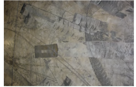
Fig. 7: Tire marks (rubber burn) on sealed concrete
