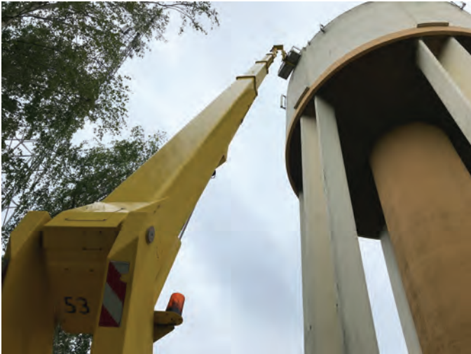
Fig. 1: First inspection from sky lift
