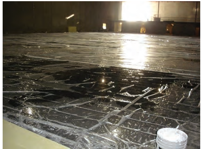
Fig. 2: Polyethylene film on green concrete
