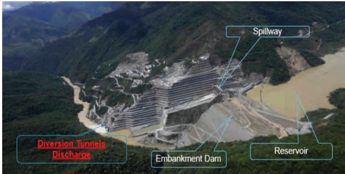
Fig. 1: The unfinished crest of the dam during the rainy season 6
