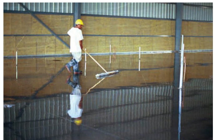
Fig. 4: Silicate application
