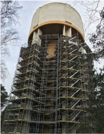
Fig. 4: Scaffolding being erected
