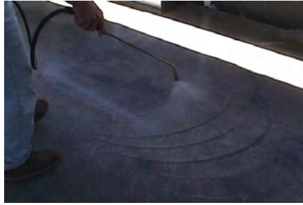
Fig. 6: Low pressure spray application of curing compound
