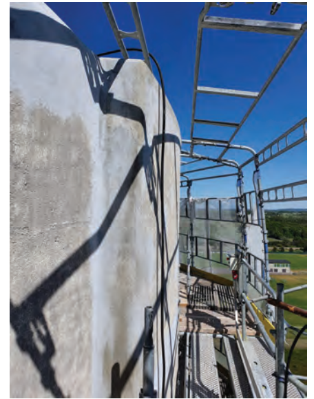
Fig. 8: Repairs on one of the upper pilasters of the reservoir
