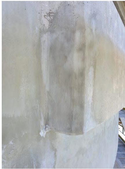
Fig. 7: Repaired area
