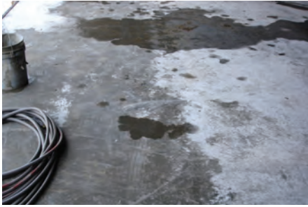
Fig. 5: Dried crystalline from over application of silicate
