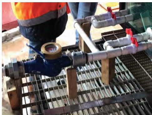
Fig. 10: Water meter used to capture the extreme water flow during the large-scale mockup in Bogota
