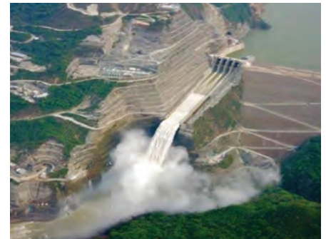
Fig. 15: The Ituango Dam spillway became operational in 2019 4
