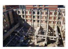
Much of the deterioration that was observed was a result of moisture infiltration into the basement and around the base of columns in the basement. Corrosion of the
