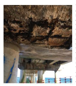
This landmark destination had suffered damage due to severe weather and heavy use. The concrete beams supporting the pressuretreated infill panels had to be repaired below the deck. To accomplish this, contractor ustom
