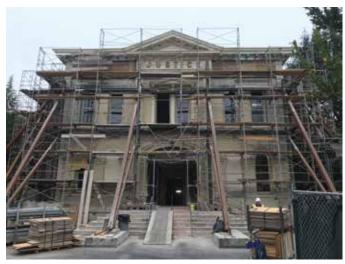
Fig. 6: The Courthouse after removing the sheathing, and prior to exterior plaster and coating work
