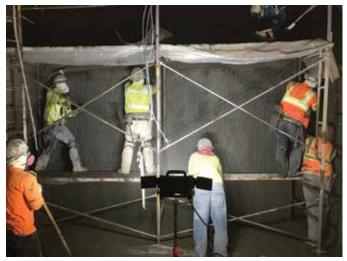
Fig. 5: Reinforcing a wall with the FRCM system
