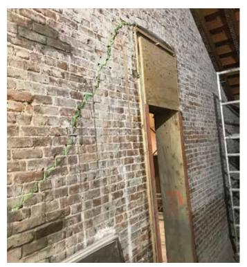
Fig. 3: Traditional masonry repair strategies, including grout injection and masonry ties, stabilized the structure to receive seismic upgrades
