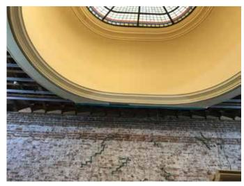
Fig. 2: The unreinforced masonry walls crumbled while the glass from the vaulted glass dome on the second floor was undamaged
