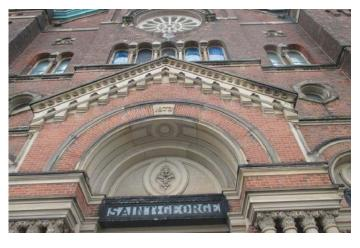
The restoration consisted of 24,000 sf (2230 sm) of exterior elevation cleaning, full re-pointing of brick masonry, stone repair, and the replacement of nearly 2,500 deteriorated bricks. Challenges included accessing the 100 ft (30 m) tall south bell towers and effectively removing the carbon buildup on the façade. A 150 ft (46 m) boom lift and citric-based gentle restoration cleaner was used to restore both
