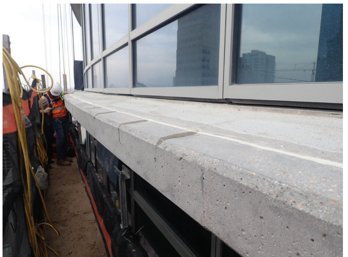
Fig. 11: Repaired slab edge after placement (note sealant joint and filled cracks)
