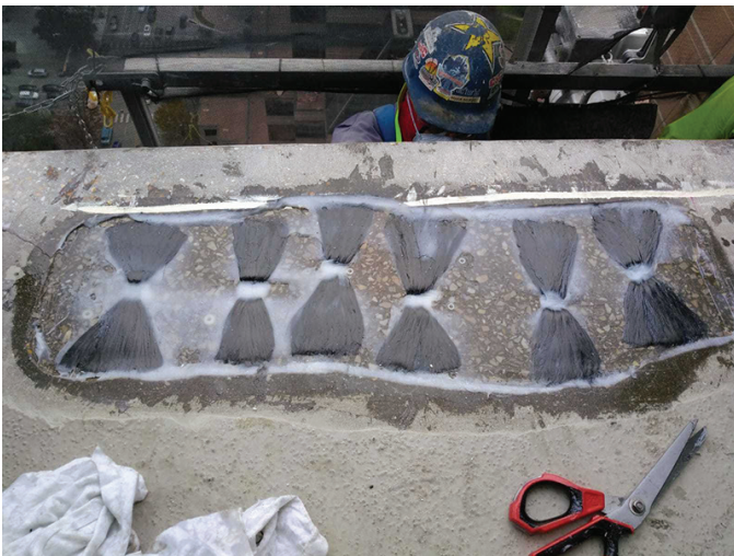
Fig. 13: Splay anchors installed to arrest existing PT bursting cracks
