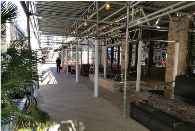
Fig. 7: Overhead protection installed around the site
