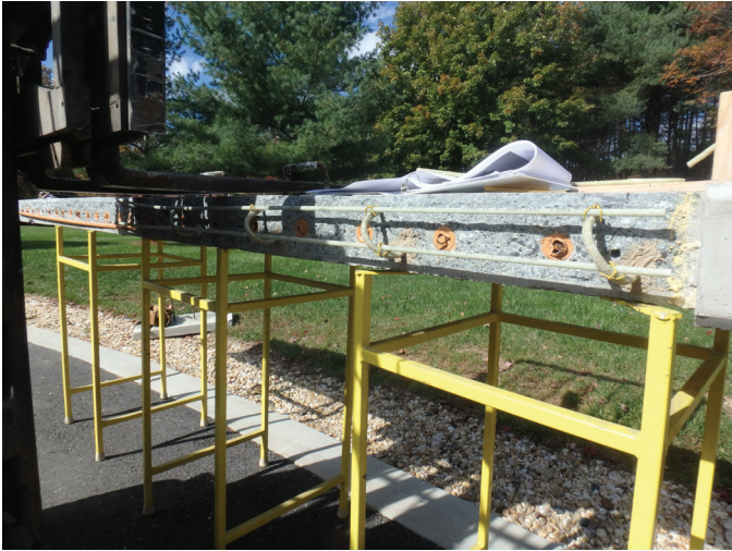
Fig. 6: Off-site mock-up showing conditions after reinforcement installation
