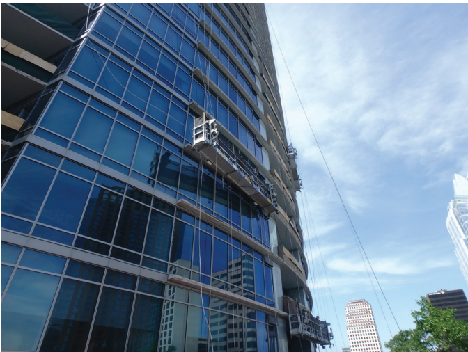
Fig. 8: Swing stages were used for access and material transportation
