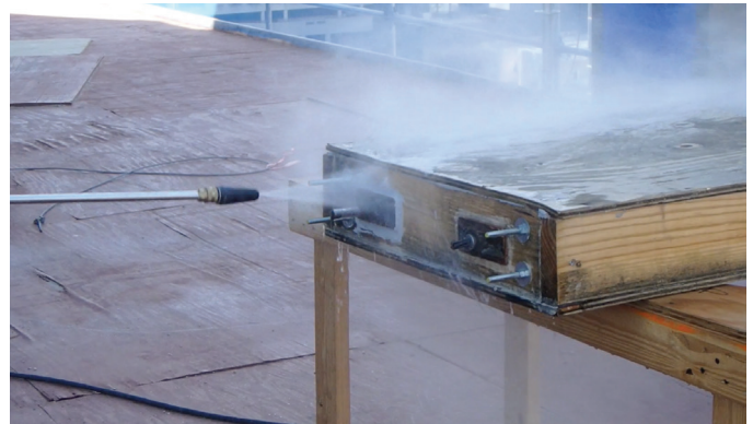
Fig. 10: Mock-up of temporary PT anchor protection
