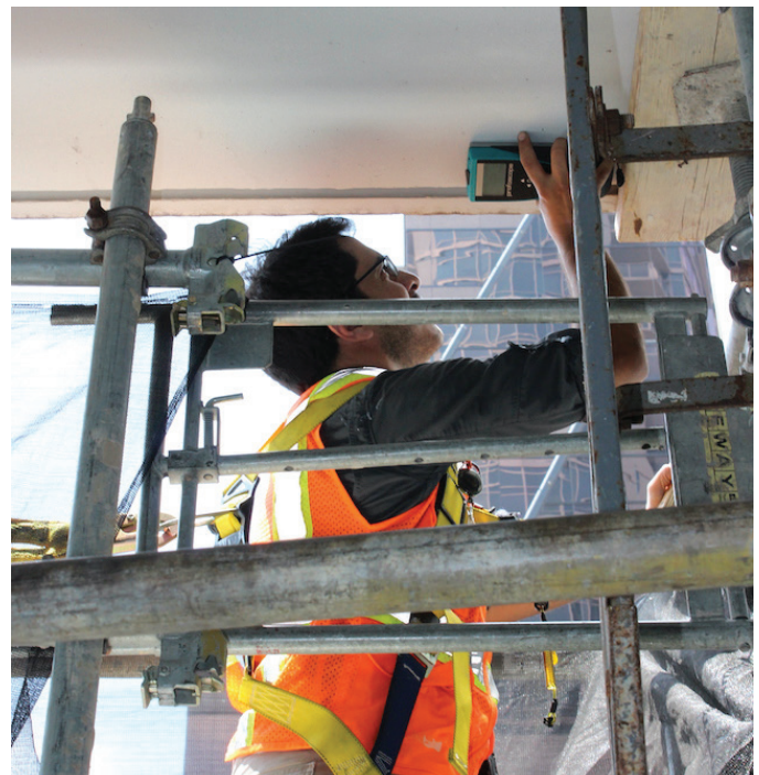
Fig. 5: Obtaining concrete cover measurements
