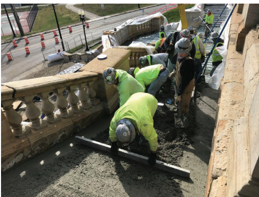
Fig. 9: Crews working on the graded slope of the grand staircase
