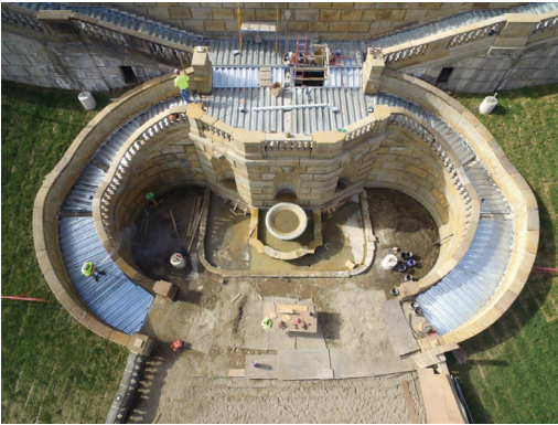
Fig. 7: Aerial view of the composite steel formwork
