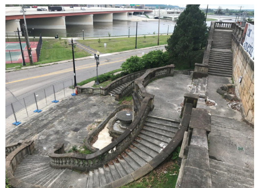
Fig. 5: Pre-construction condemned staircase
