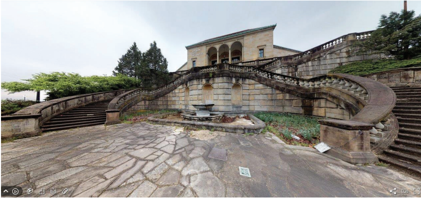
Fig. 6: 3-D scan of the grand staircase prior to construction
