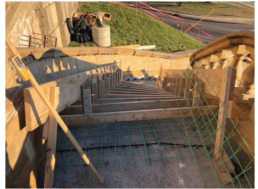
Fig. 10: Detailed formwork and anchoring
