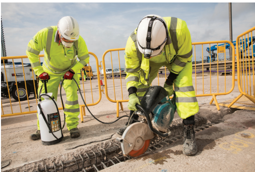
Fig. 7: Saw-cutting edges for concrete repair
