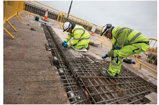
Fig. 9: Installation of embedded galvanic anodes
