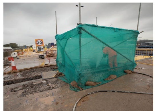
Fig. 5: Hydrodemolition of the concrete
