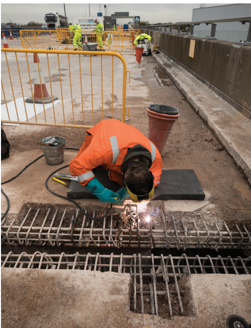
Fig. 8: Welding in new reinforcement steel
