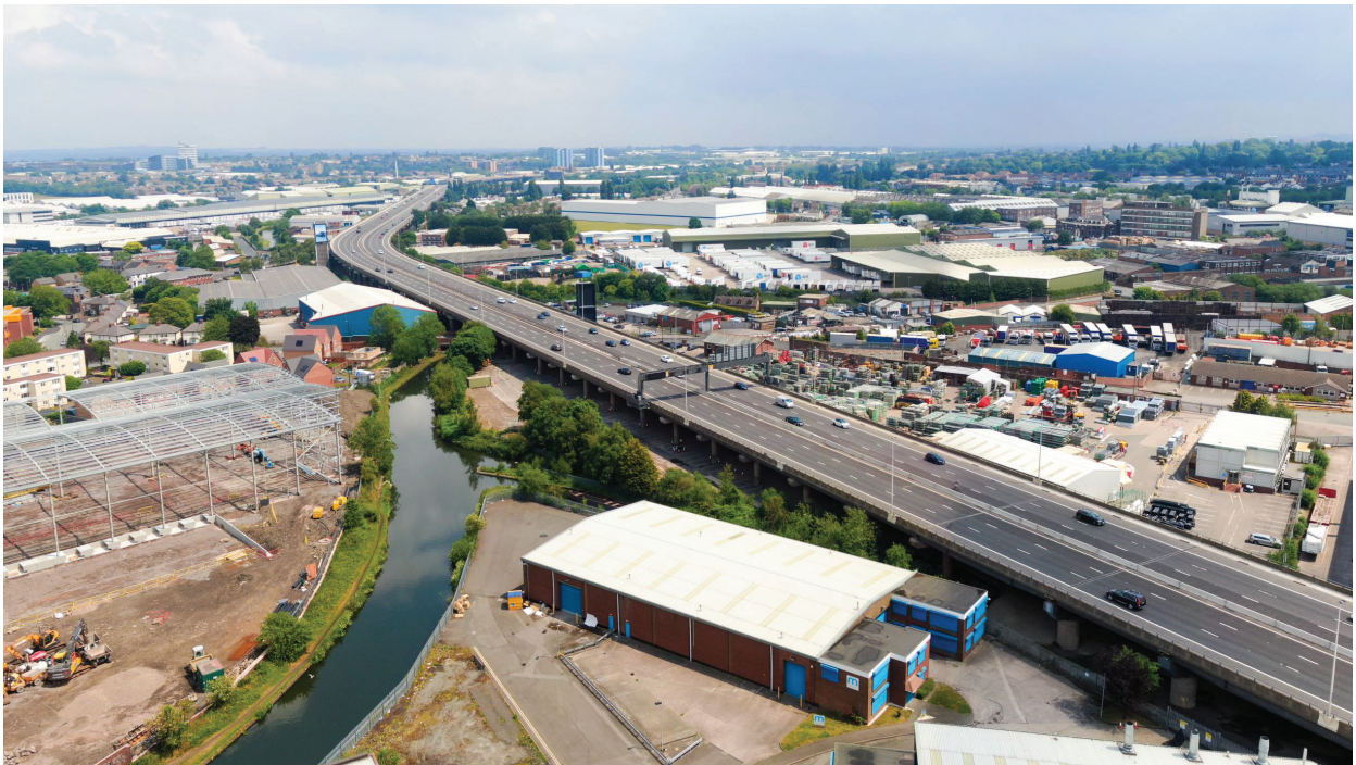
Fig. 1: Overhead view of M5 Oldbury Viaduct
