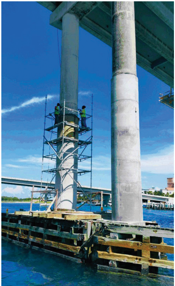
Fig. 3: Repair work at one of the columns
