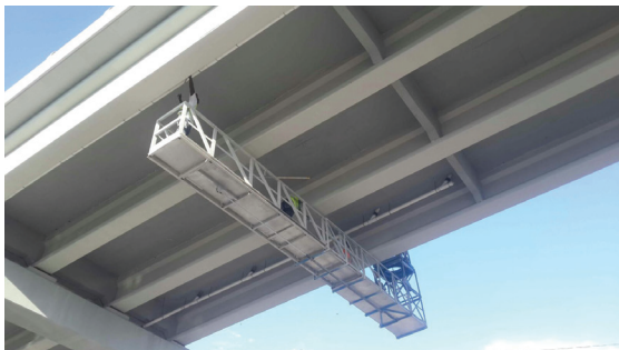
Fig. 6: Protective coating installation at bridge underside
