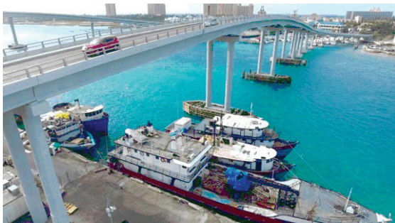
Fig. 7: Completed repairs at East Bridge
