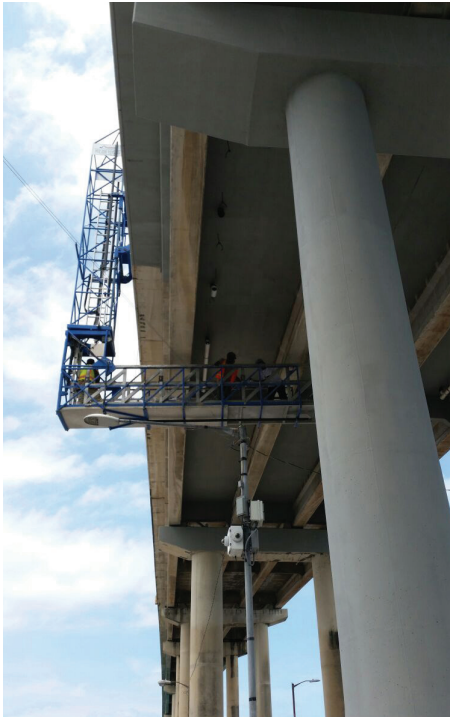
Fig. 4: Swinging platform to perform spall repairs and apply coating
