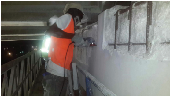
Fig. 5: Concrete repairs performed from swinging platform
