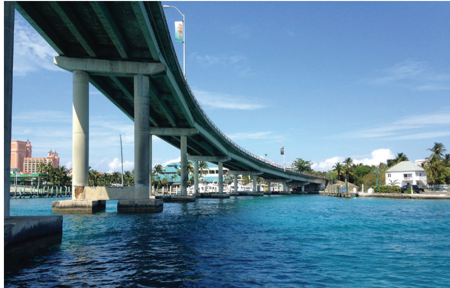
Fig. 1: East Bridge connects Nassau and Paradise Island
