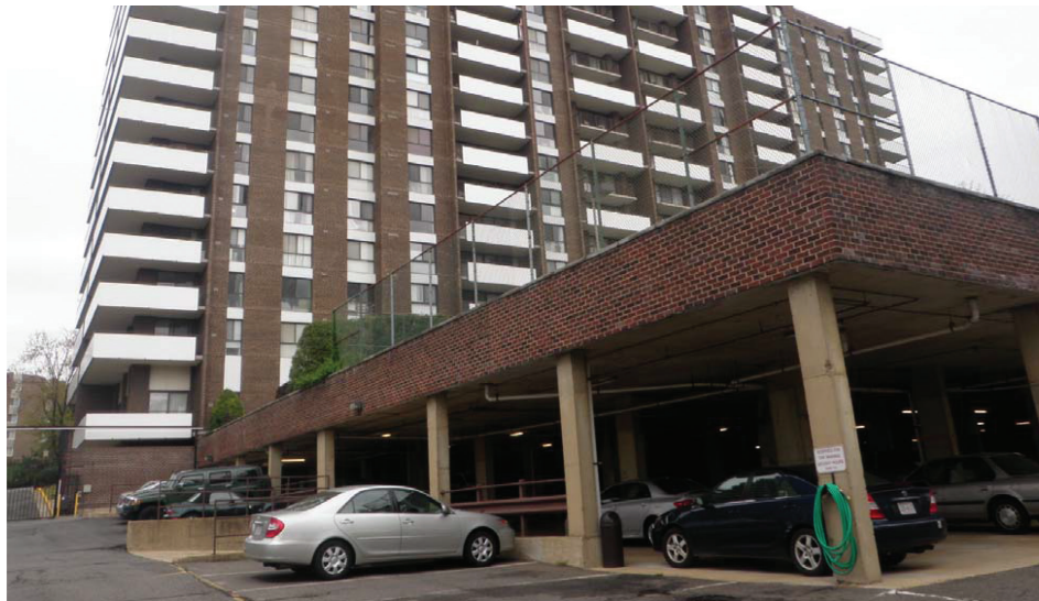
Fig. 1: Condominium building and elevated plaza structure over the garage
