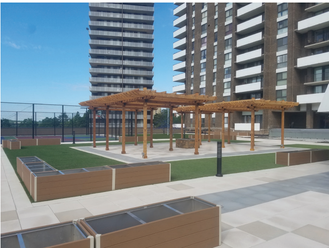
Fig. 8: Completed amenity space with hardscaping
