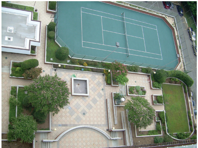
Fig. 2: Bird's eye view of the plaza (planters, pavers, soil and hardscaping)
