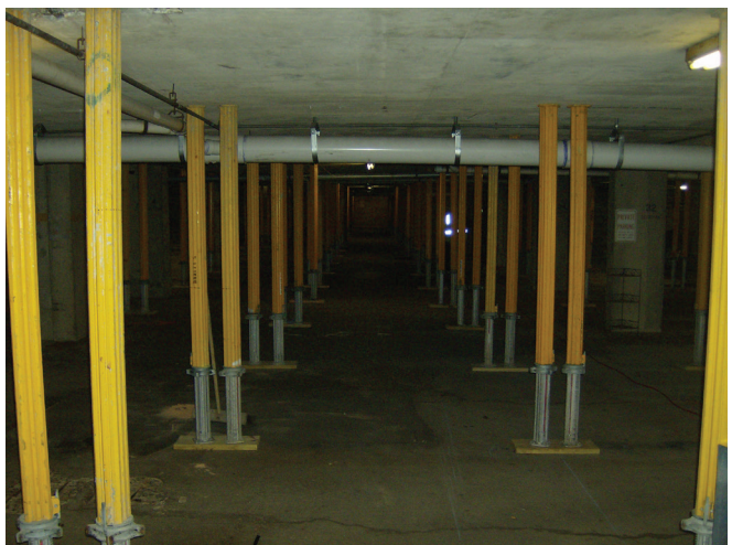
Fig. 4: Shoring for plaza during the emergency load reduction phase
