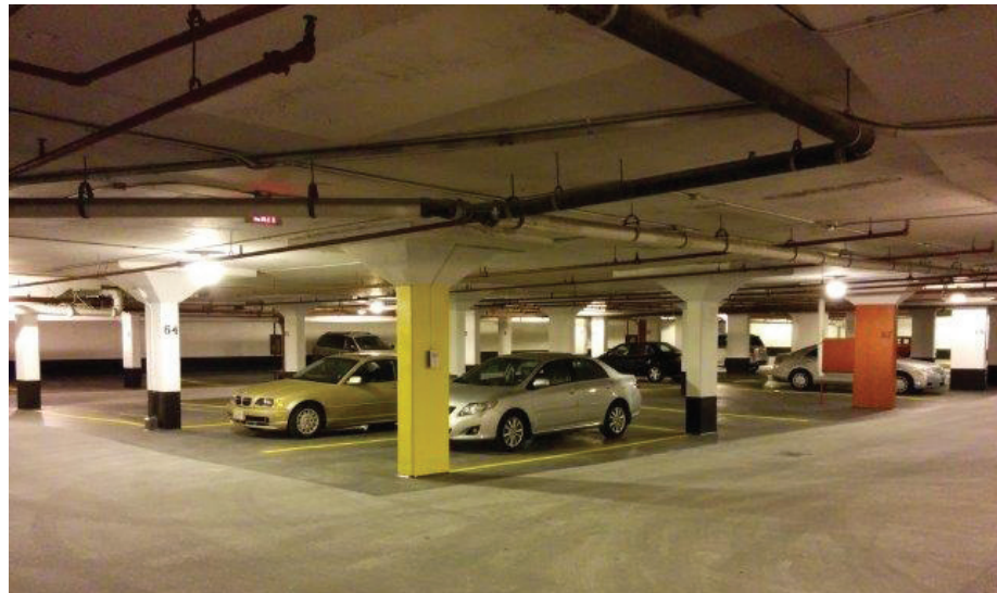
Underground parking garage structure at 275 Bamburgh Circle in Markham, Ontario.
