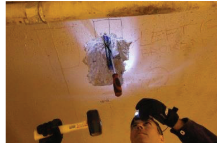
Fig. 2: Penetration testing on PT cable
