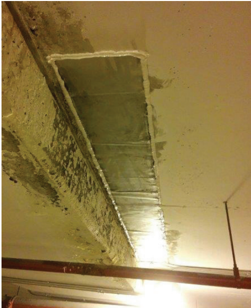
Fig. 7: Sacrificial zinc sheet at slab soffit
