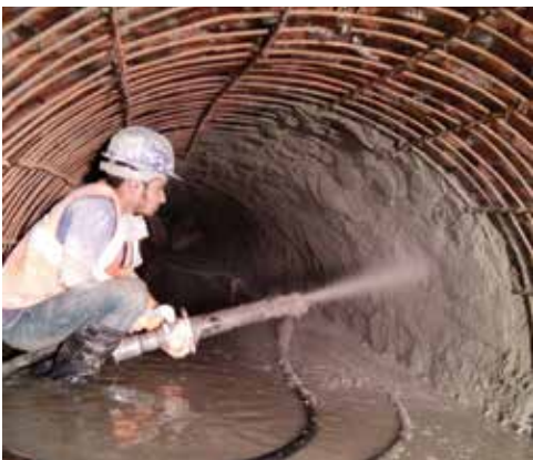
Fig. 9: Installing wet-mix shotcrete
