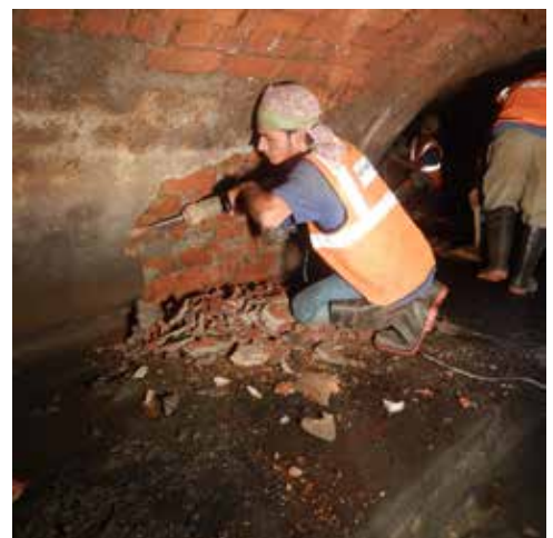
Fig. 5: Demolition of deteriorated brick lining with lightweight breaker
