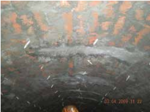
Fig. 7: Installed ports for injecting 2-component rigid polyurethane resin
