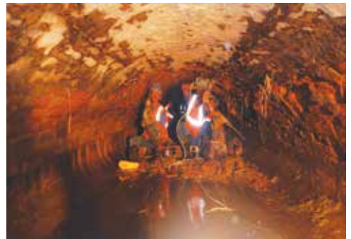
Fig. 4: Root penetration
