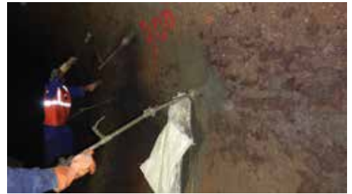
Fig. 11: Fixing packers and grouting using a non-shrink cementitious, anti-washout grout
