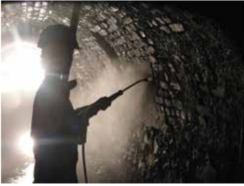
Fig. 6: High-pressure waterjet washing
