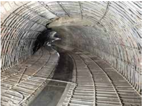
Fig. 8: Fixing reinforcement FE 500D
