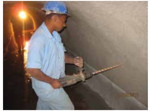
Fig. 10: Drilling holes into the brick masonry
