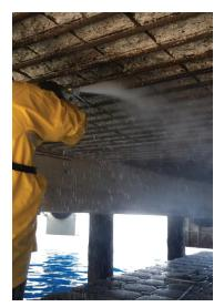
The repair program included the following items: Cementbased rustproofing, with migrating corrosion inhibitor, was applied to protect steel surfaces. Deteriorated concrete was
