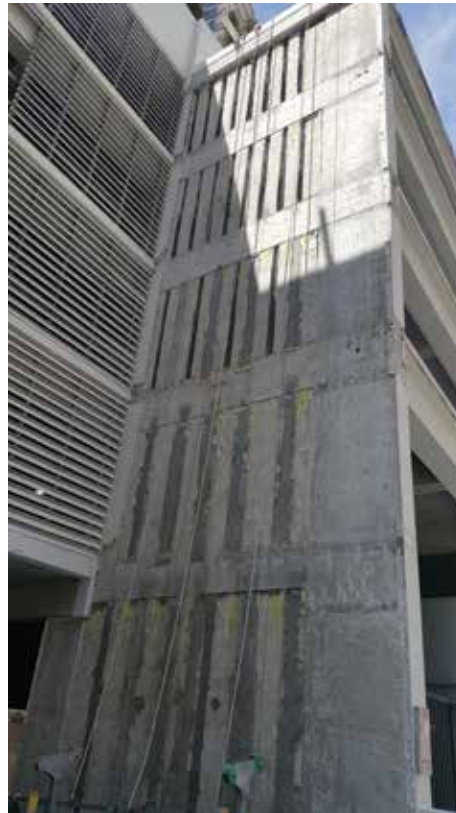
Fig. 7: Parking garage shear wall/barrier wall being reinforced
