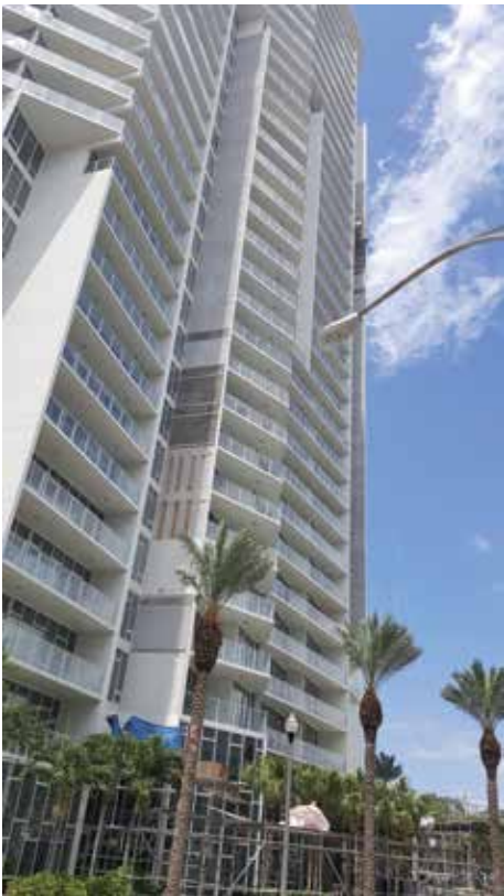
Fig. 6: Shear wall under various phases of repair
