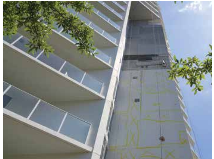
Fig. 3: Stucco marked up for removal after sounding
