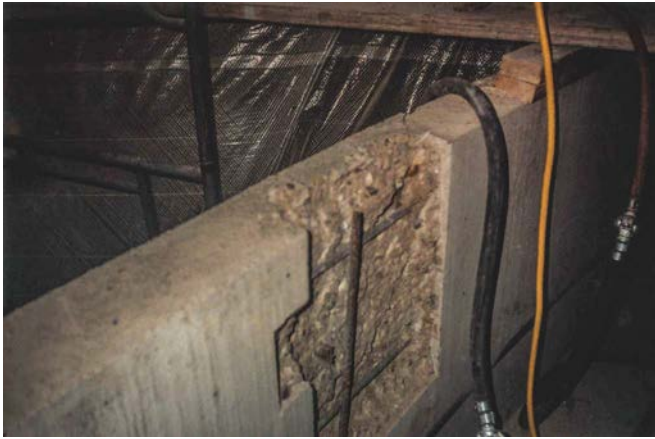
Fig. 8: Knee wall vertical repair demolition
