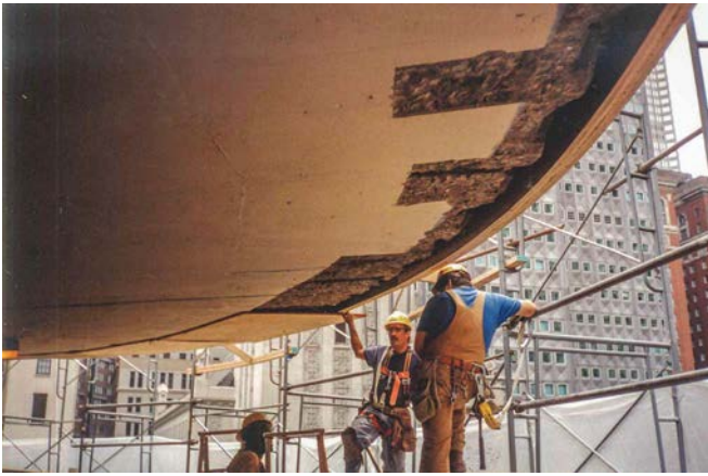
Fig. 5: Slab edge soffit demolition and formwork
