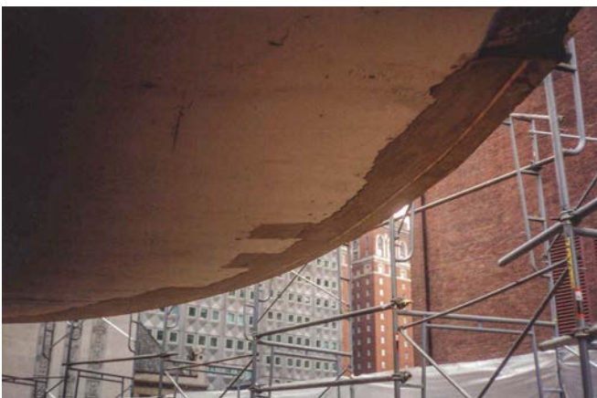
Fig. 7. Completed slab soffit repair with integral drip edge
