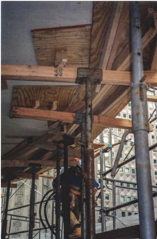
Fig. 6: Slab edge formwork and shoring
