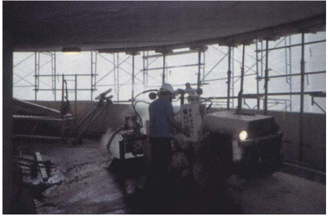
Fig. 9: Hydrodemolition of upper concrete layer at ramp slab
