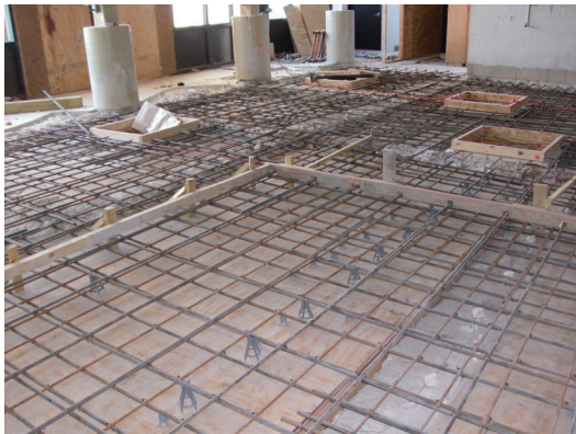
Fig. 5: New slab formed with new reinforcing steel
