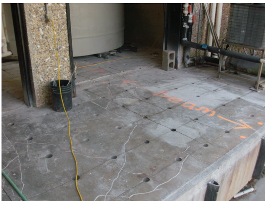
Fig. 6: Core holes and slots for galvanic protection in Lab B, 2010
