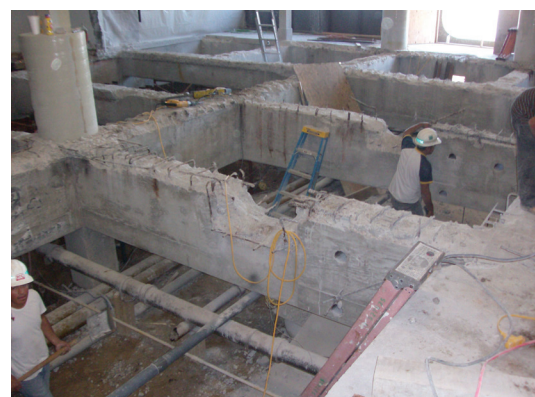
Fig. 4: Demolition at Lab A
