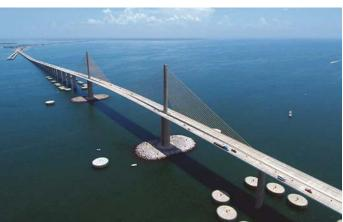
The Sunshine Skyway Bridge is comprised of the main span, the high level approach, and the low level trestle spans. Shear cracking was observed during routine inspections of the trestle span girders. Repairs included epoxy injection of all cracks having a width exceeding 0.012 in (0.3 mm), repairing spalls, and filling uneven surfaces with a leveling mortar and all bugholes and smaller cavities with an epoxy paste. A clear protective sealer was applied to protect the concrete further from
