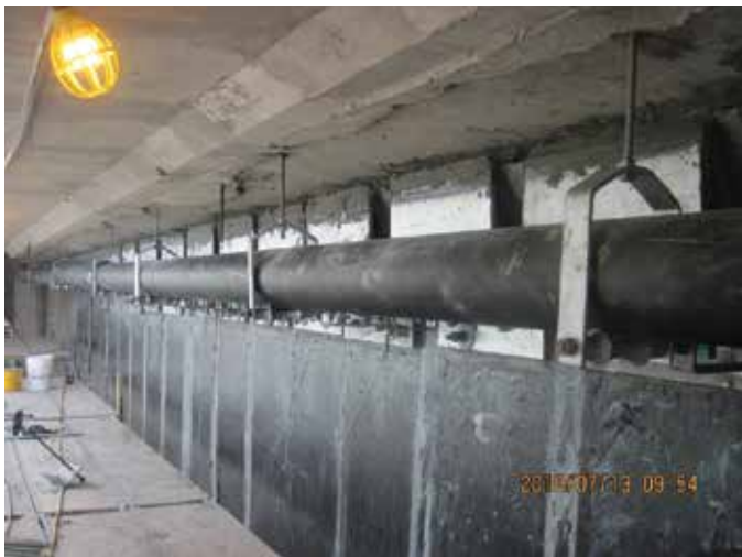
Fig. 14: External post-tensioning system
