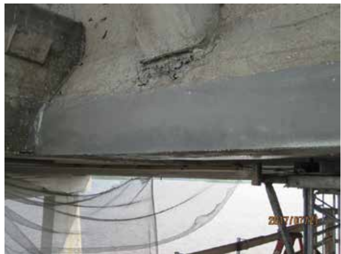
Fig. 6: Repaired girder using mortar concrete
