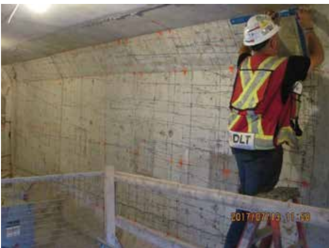
Fig. 4: Rebar and strand identification
