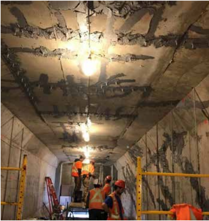
Fig. 8: Crack injection preparation
