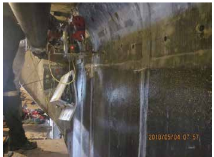
Fig. 13: Installed CFRP strips
