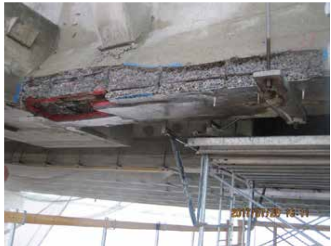
Fig. 5: Typical lower flange girder concrete demolition
