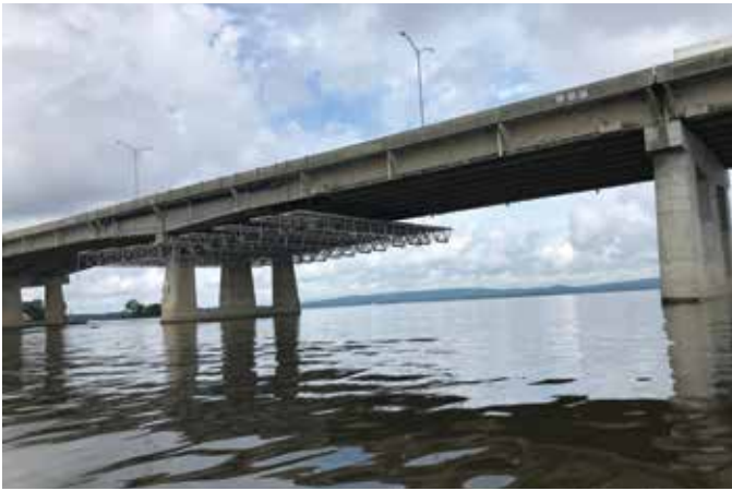
Fig. 2: Working platforms over the maritime corridor
