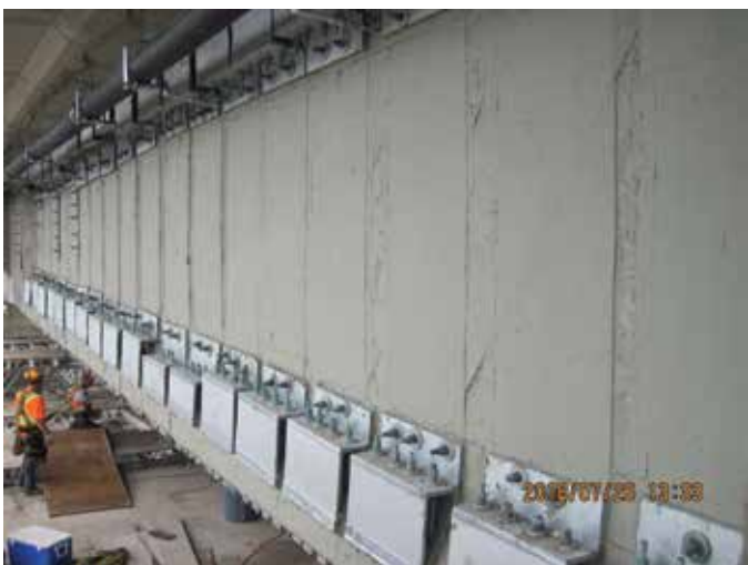
Fig. 15: External view of girder after completion of work
