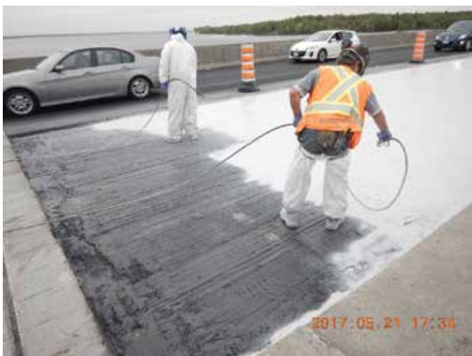
Fig. 16: Spray applied waterproofing deck membrane application
