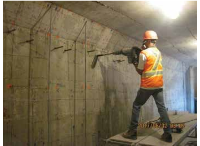
Fig. 9: Steel CFRP anchor plate horizontal hole drilling
