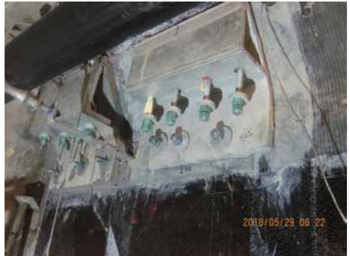
Fig. 12: Steel CFRP anchor plates
