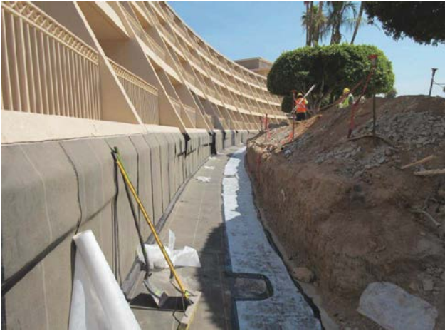
Fig. 6: New membrane and flashing along the expansion joint and building wall
