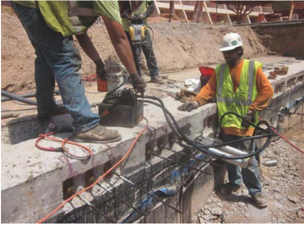
Fig. 5: Post-tension repairs in progress (stressing end)
