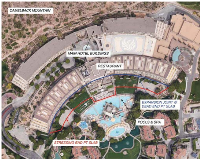
Fig. 2: Overhead view of subgrade garage
