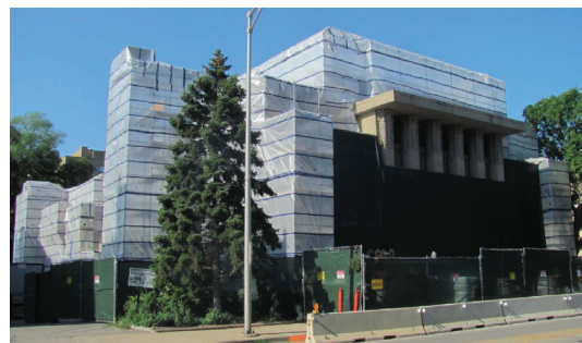
Fig. 5: Weather enclosure at front (north) elevation of Unity Temple during restoration
