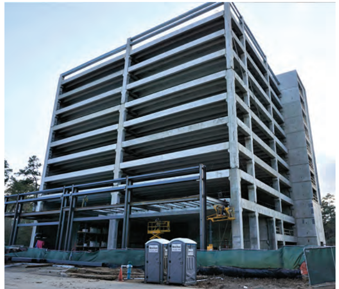
Fig. 4: 11-story precast structure
