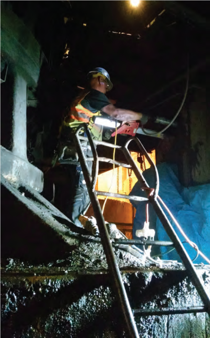
Fig. 5: Coring operation at side of column
