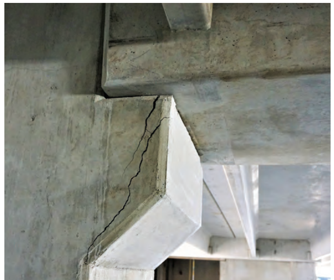
Fig. 5: Corbel cracking
