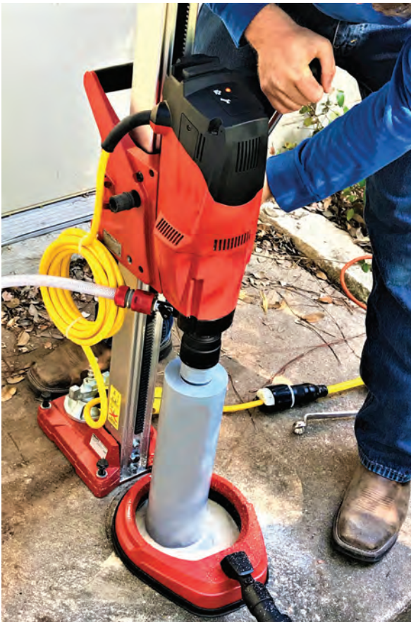
Fig. 3: Concrete coring
