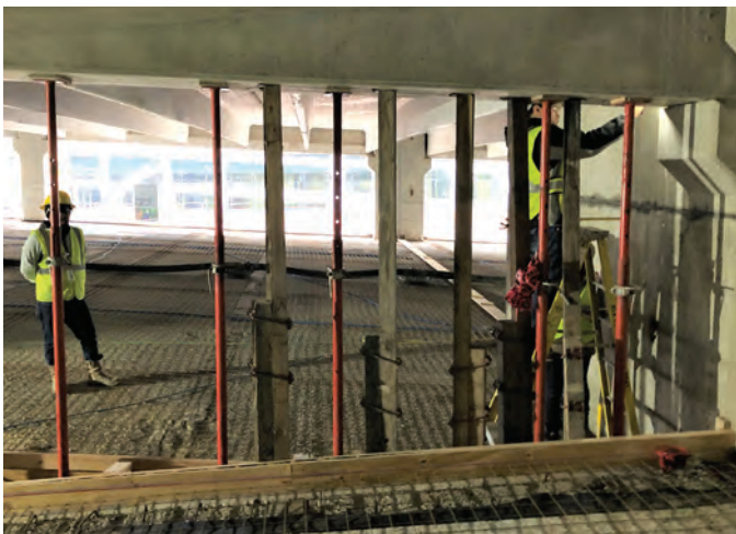
Fig. 7: Shoring of L-shaped girder
