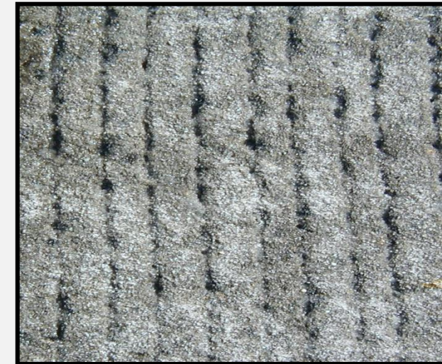
When cured, remove excess sand and open to traffic
