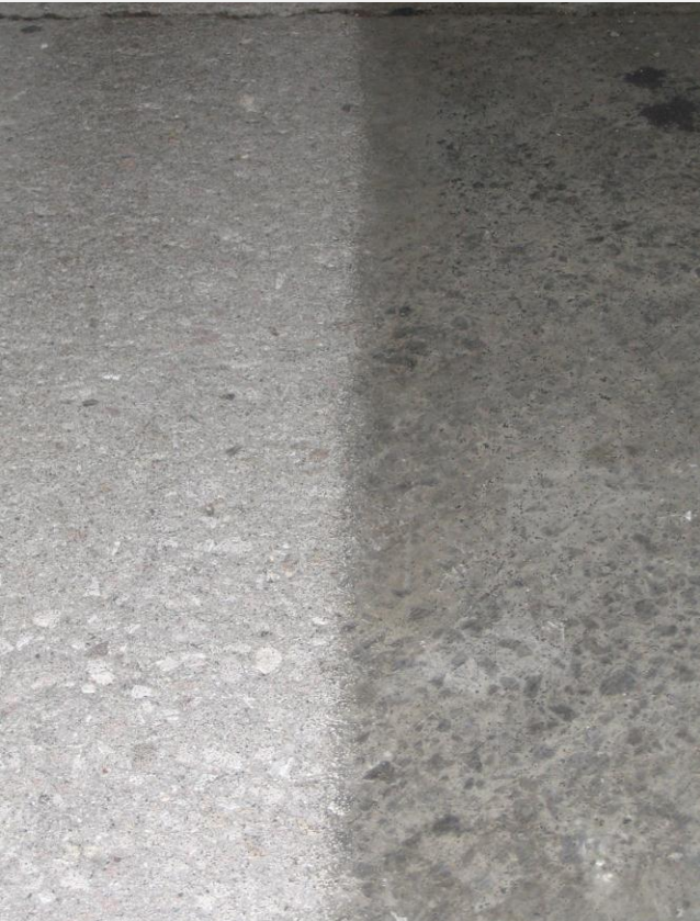
Steel Bead Blasting
