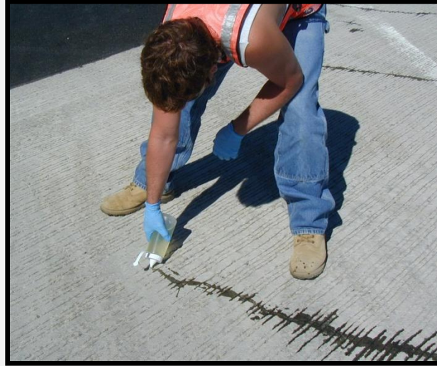
Pre-treat larger cracks if necessary
