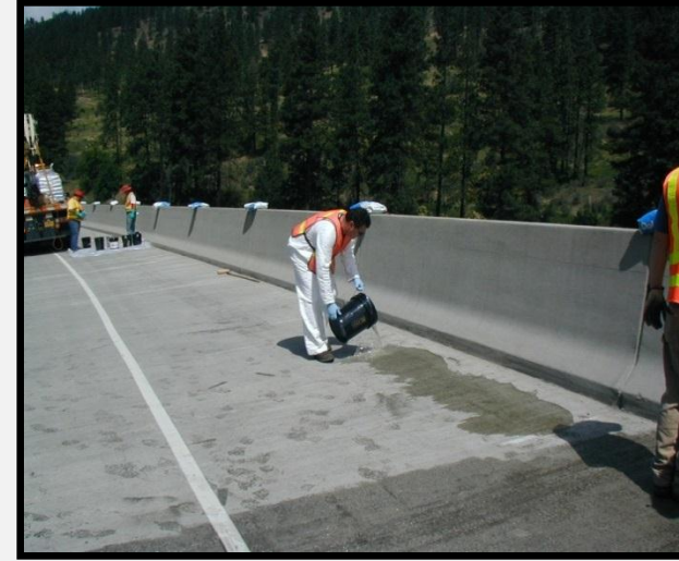
Flood surface with properly mixed epoxy
