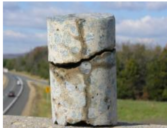
C5 – delamination at 2.5 inches
