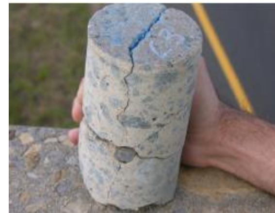
C3 – delamination at 3.5 inches
