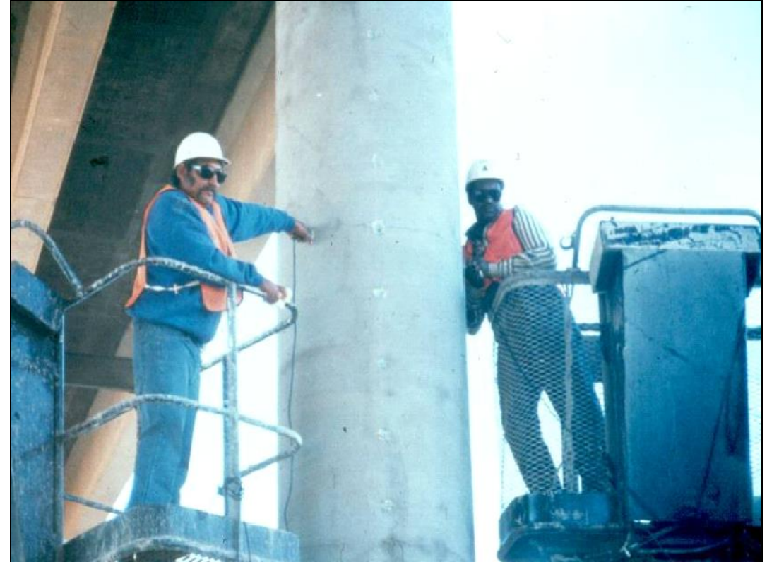
UPV Testing on a Column
