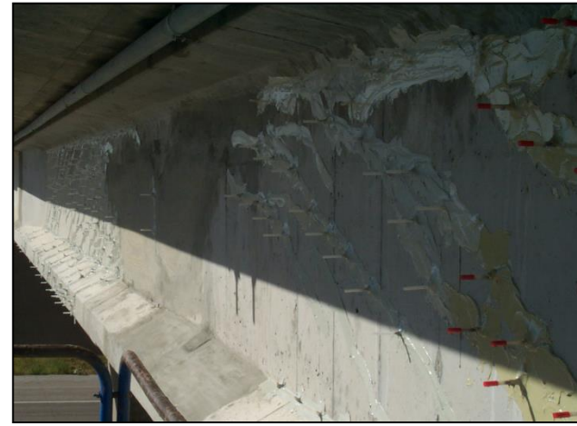
Epoxy Injection for Crack Repairs
